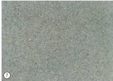
⑦ Concrete Paving At Stoops
