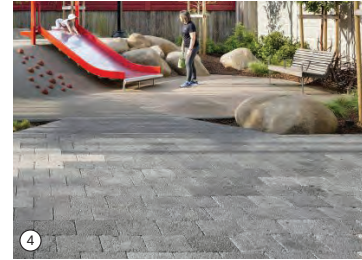
④ Permeable Paving Banding
