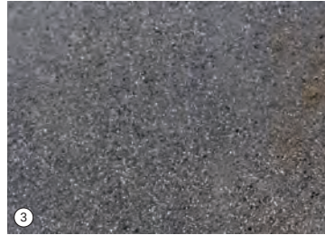
③ Integral Color Concrete Banding
