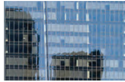
Block 5 - Park Tower
