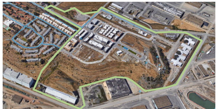
Figure 2 Aerial view of Parcel A-1
