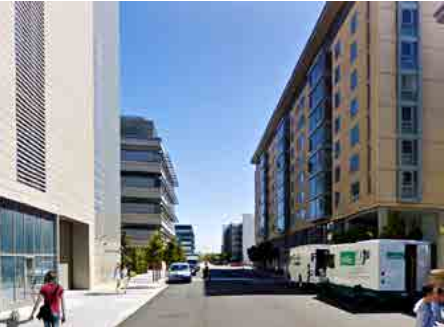
Current Pierpoint Lane: View toward the Bay.
