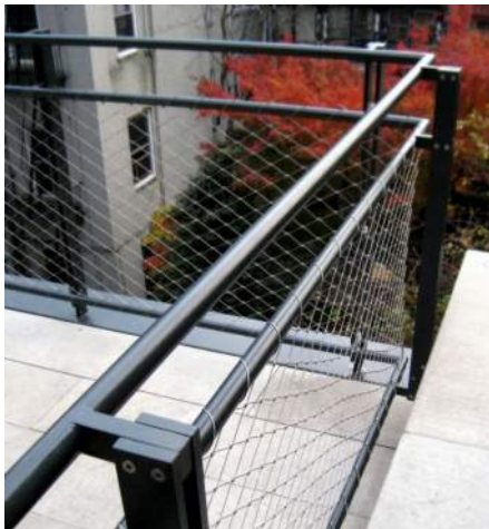
(R5) Guardrail/Bar Rail/Counter Custom painted steel rail and bar counter space with inset stainless steel mesh panels - Jakob Rope Systems "Webnet" or similar
