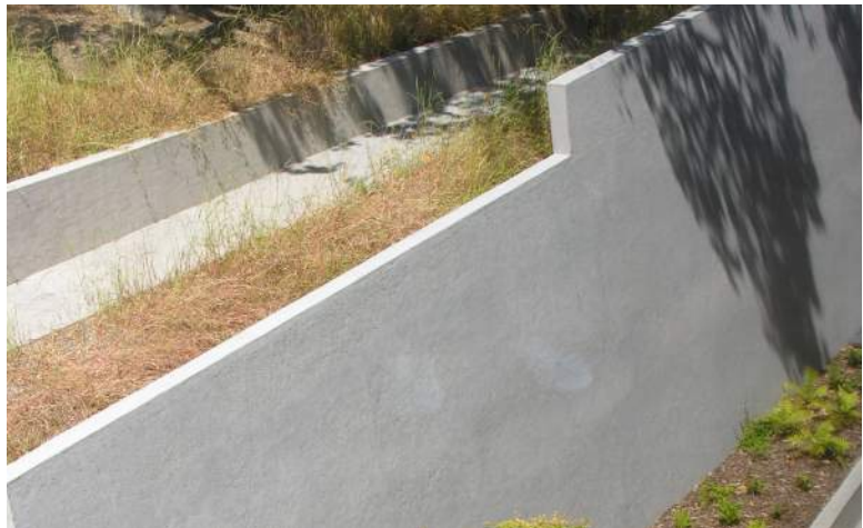
(R7) Retaining Walls CIP architectural concrete with light sandblast finish
