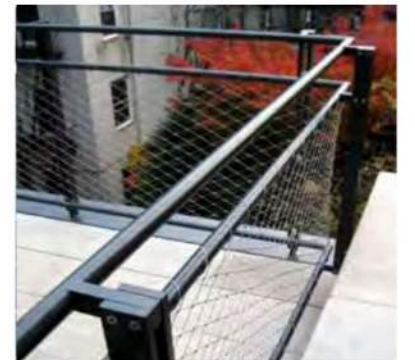
06 Stainless Steel Cable Mesh Gaurdrail (See Page 61)
