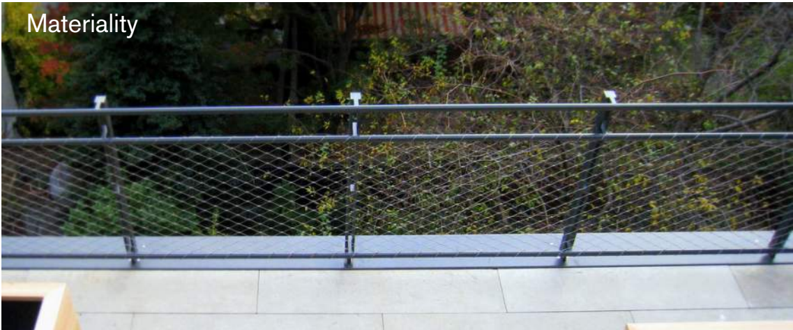
(R3) Dog Park Fence and Gate Custom painted steel with inset stainless steel mesh panels - Jakob Rope Systems "Webnet" or similar
