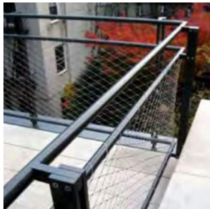
Stainless Steel Cable Mesh Guardrail (See Page 61)
