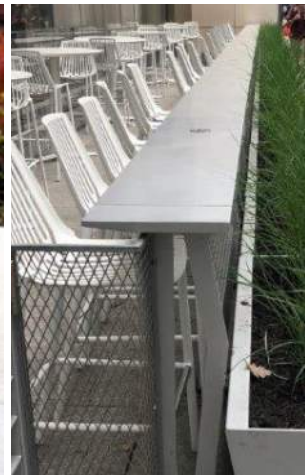
(R5) Guardrail/Bar Rail/Counter Custom painted steel rail and bar counter space with inset stainless steel mesh panels - Jakob Rope Systems "Webnet" or similar
