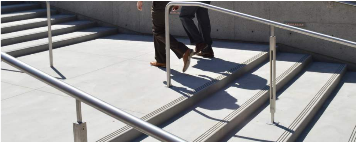
(R1) (R2) Stair and Ramp With Handrails
