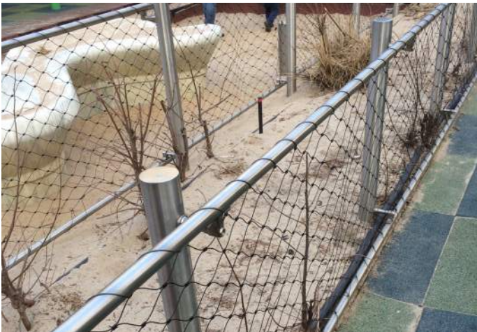
(R4) Dog Park Low Fence at Planting Custom steel barrier fence with inset stainless steel mesh panels - Jakob Rope Systems "Webnet" or similar
