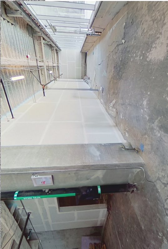
PHOTO EXISTING CONDITIONS TMM MAIN ENTRANCE PROPOSED WALL WRAP BANNER
