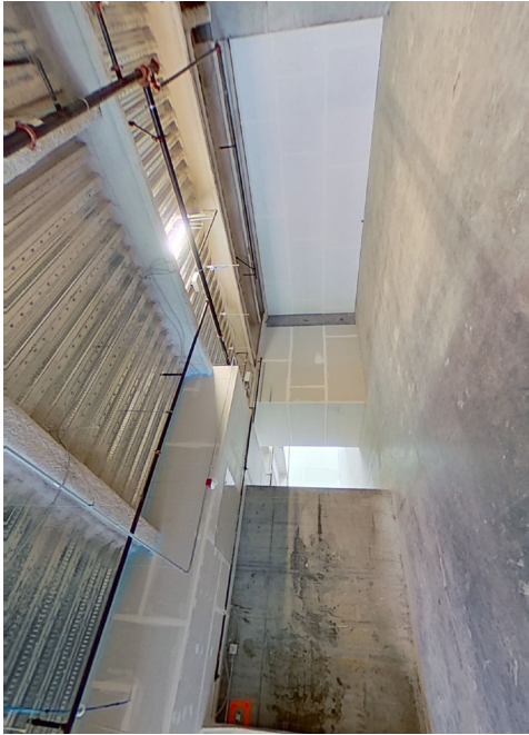
PHOTO EXISTING CONDITIONS
