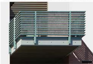
METAL BALCONY & GUARDRAIL WITH DENSE MESH BACKING
