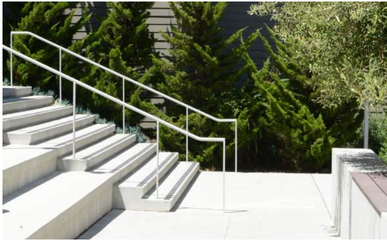
10 HANDRAILS AT RAMPS PRIMED & PAINTED GALVANIZED STEEL
