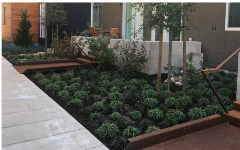
③ FLUSH STORMWATER PLANTER WITH 6" PONDING AREA
