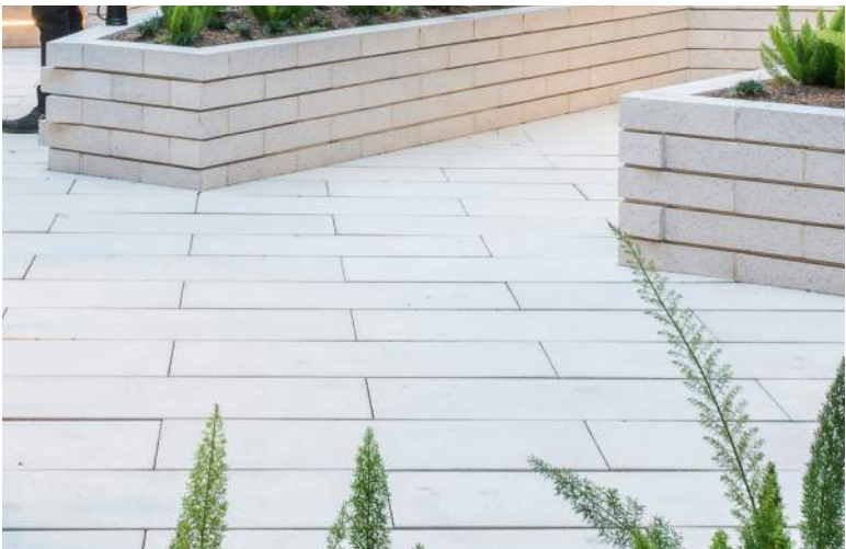
12 1'x3' UNIT PAVERS AT UPPER COURTYARD
