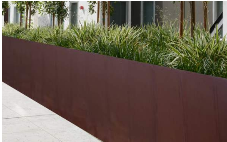
② RAISED STORMWATER PLANTER CORTEN STEEL
