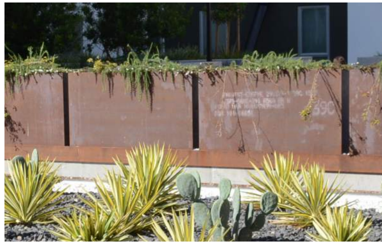
15 PLANTED EDGE PROTECTION 42" HIGH CORTEN STEEL
