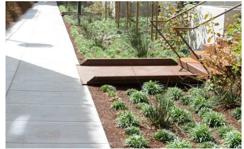
18 HINGE BRIDGE OVER MEWS PLANTERS CORTEN STEEL
