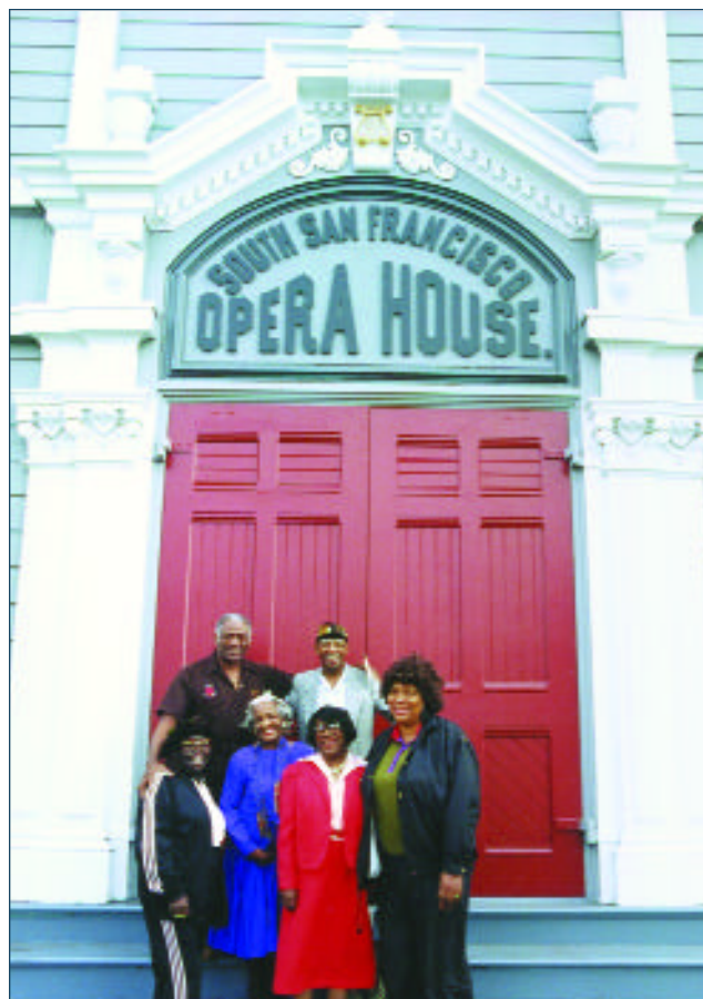
Designated Landmark No. 8 by the City and County of San Francisco, the Opera House is the sole surviving theatre of pre-fire San Francisco. Courtesy Bayview Opera House Ruth Williams Memorial Theatre.
