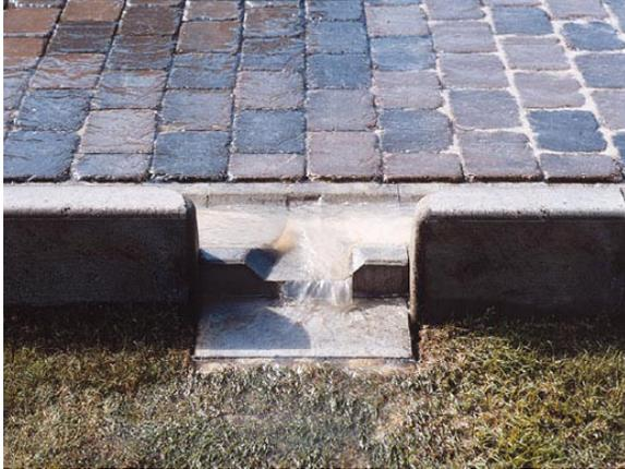
*Slotted curbs allow surface runoff into swales*
