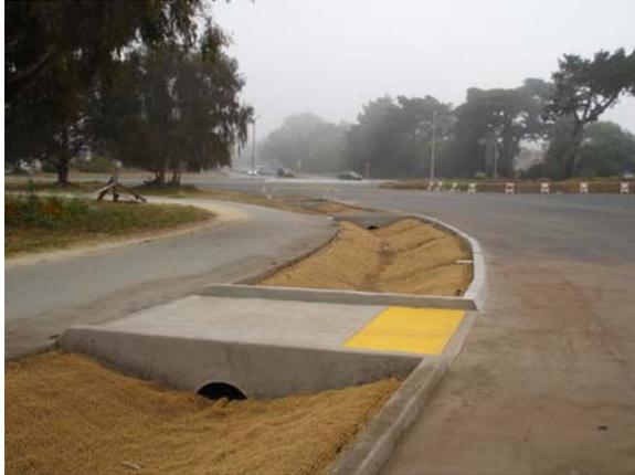
*“Sunset Swales,” SFPUC demonstration project, during construction*
