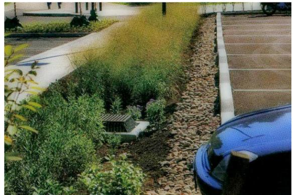
*Bio-retention filter strip and swale*
