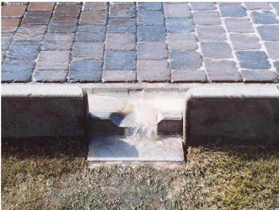
*Slotted curbs allow surface runoff into swales*
