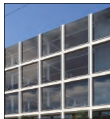
STRUCTURAL STEEL/ CURTAIN WALLS
