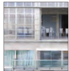
GLASS Façade/ CONCRETED STRUCTURE
