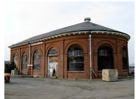
Pumphouse at Drydock 3
