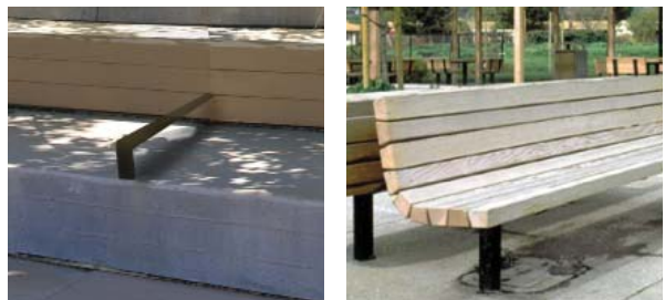
03 C.I.P. Concrete Seat-wall w/ Back 04 Wood Bench w/ Steel Frame
