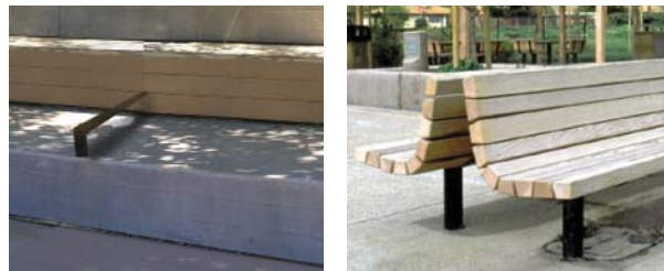
03 C.I.P. Concrete Seat-wall with Back 04 Wood Bench w/ Steel Frame
