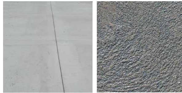
① C.I.P. Concrete Paving ② C.I.P. Concrete Paving
