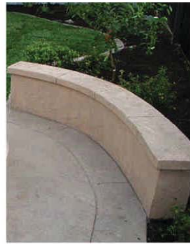
C.I.P. Concrete Seatwall
