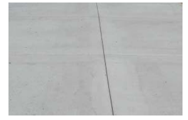
A C.I.P. Concrete Paving
