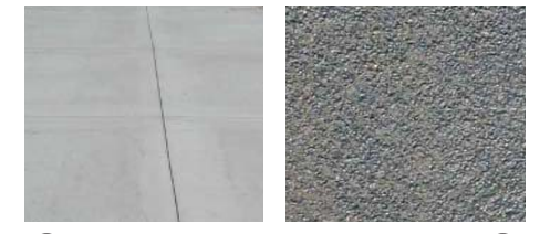
A C.I.P. Concrete Paving
