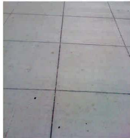
C.I.P. Concrete Paving
