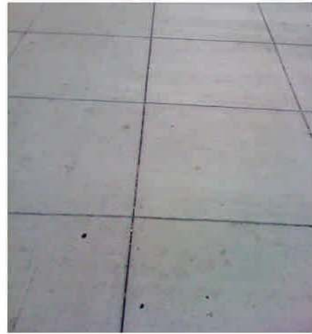
C.I.P. Concrete Paving
