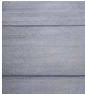
01 C.I.P. Concrete Paving
