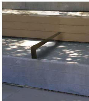
04 C.I.P. Concrete Seatwall w/ Back
