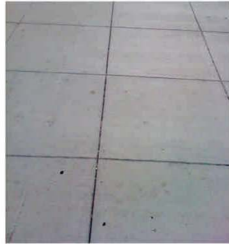
C.I.P. Concrete Paving
