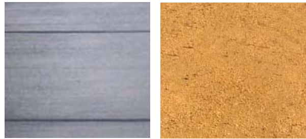
01 C.I.P. Concrete Paving 02 Stabilized Crushed Stone Paving
