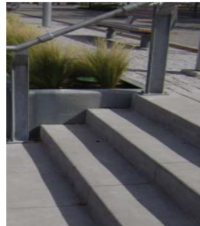
02 C.I.P. Concrete Stair w/ Metal Handrail
