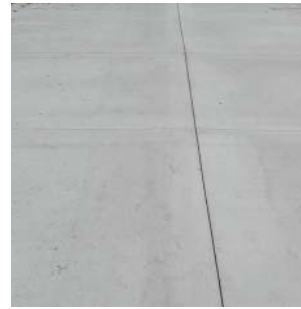
① C.I.P. Concrete Paving
