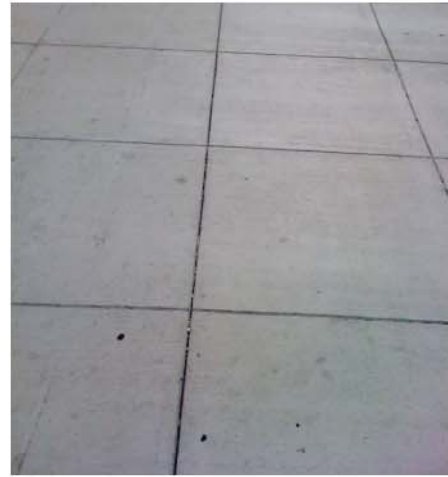
C.I.P. Concrete Paving
