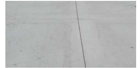
A C.I.P. Concrete Paving
