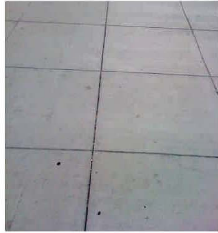
C.I.P. Concrete Paving
