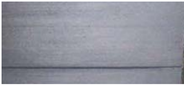
01 C.I.P. Concrete Paving
