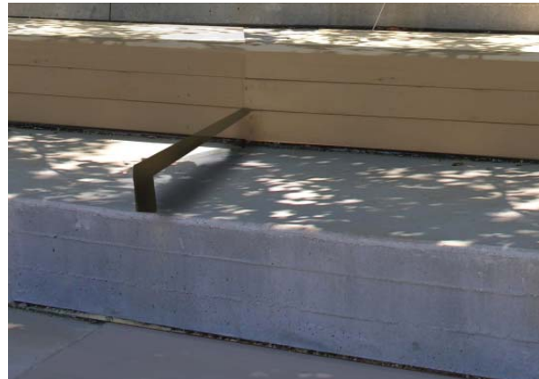
03 C.I.P. Concrete Seat-wall w/ Back
