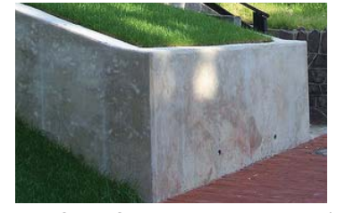
B C.I.P. Concrete retaining wall/ Seatwall
