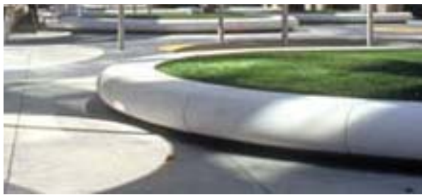
03 C.I.P. Concrete Seatwall / Planter
