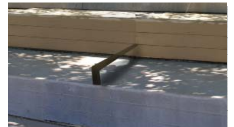
B C.I.P. Concrete Seatwall with Back
