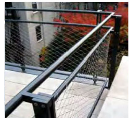
06 Stainless Steel Cable Mesh Gaurdrail (See Page 61)
