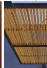
Metal & Wood Awning
