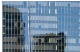
Block 5 - Park Tower
