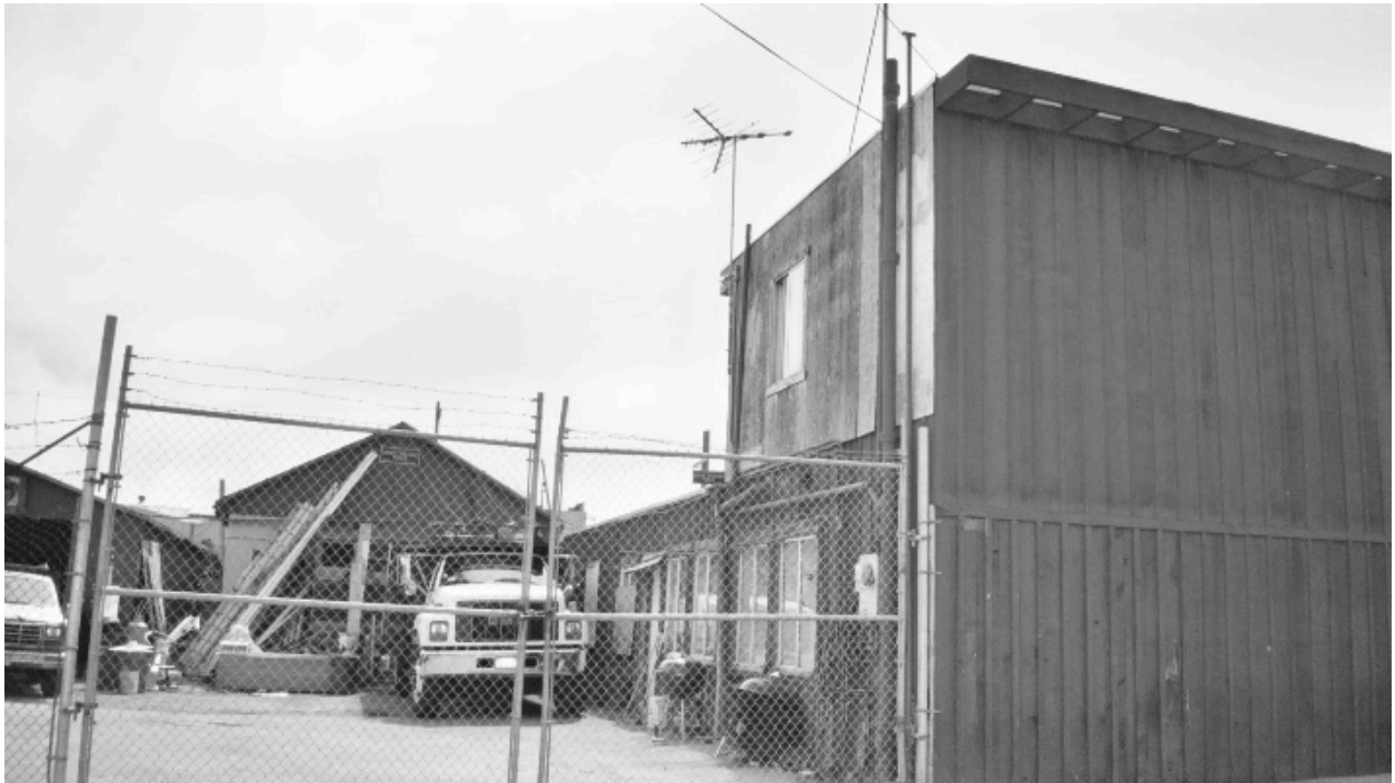
2105 Keith Street: Dilapidated building (on the right), deteriorated siding and trim, peeling paint, boarded window, trash accumulation and outside storage.
