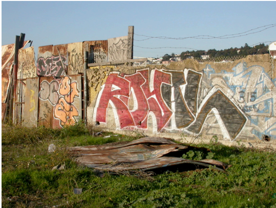
Wallace Avenue between Ingalls Street and Hawes Street: Unpaved street, trash accumulation, informal and substandard construction of fences, graffiti.
