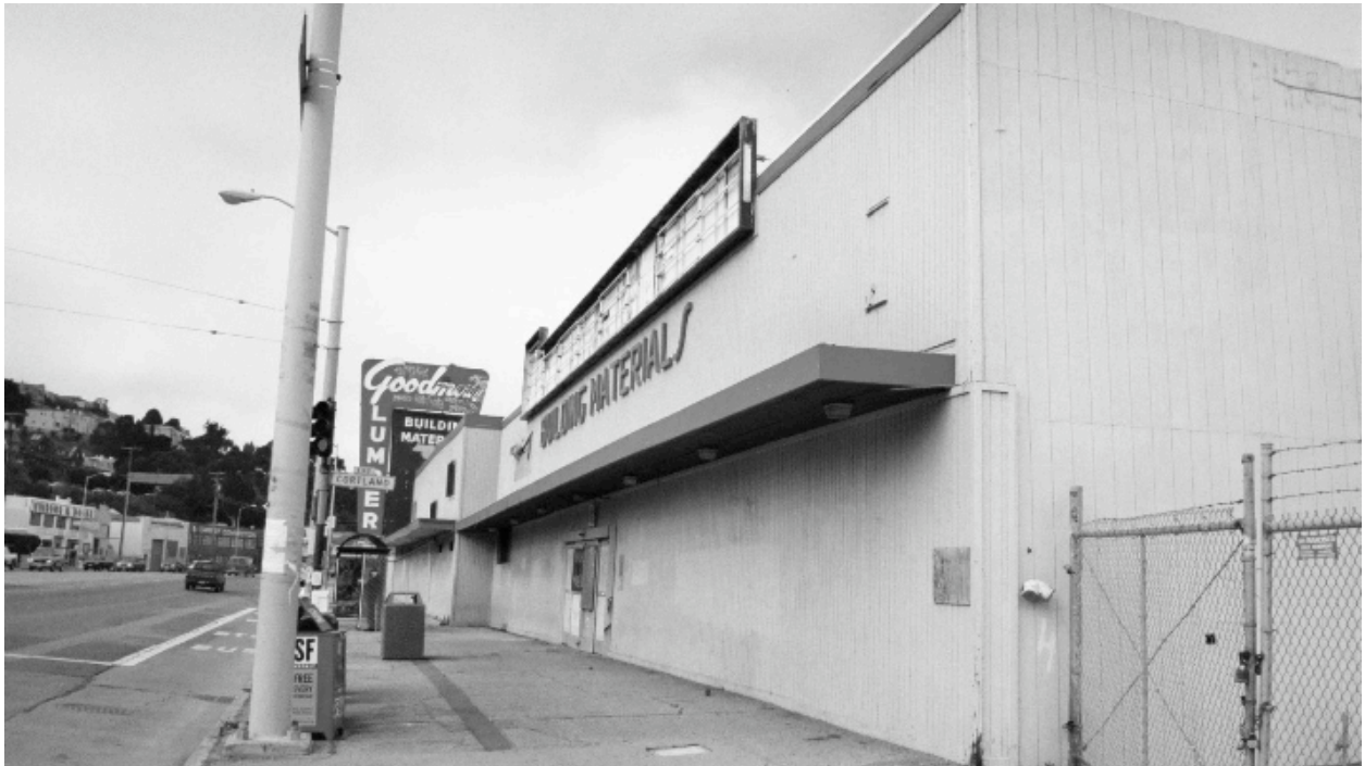
East side of Bayshore Boulevard at Cortland Avenue: Large, vacant deteriorated building formerly Goodman's Lumber, deteriorated signage and siding, broken windows, boarded windows and doors, deferred maintenance, sagging overhang, graffiti, cracks and holes in sidewalk.
