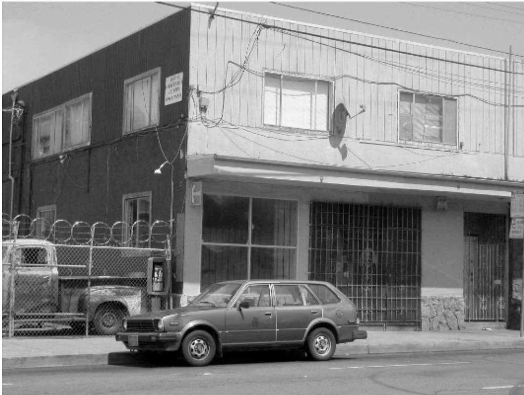
994-998 Gilman Street: Extensively deteriorated building; deteriorated siding, paint and windows; faulty wiring. Former commercial storefronts apparently being used as residences.
