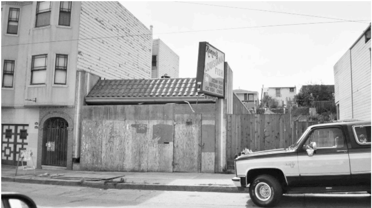
5286 Third Street: Vacant, boarded up, extensively deteriorated building, deteriorated siding and signage.
