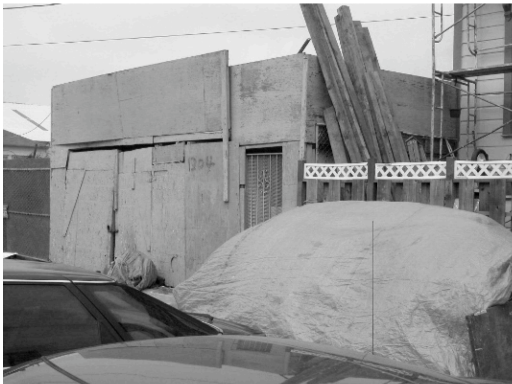
1304 Egbert Avenue: Dilapidated garage, informal construction, deferred maintenance, deteriorated siding, accumulated trash and storage on sidewalk.
