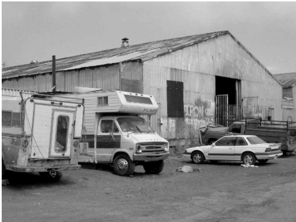
1230 Underwood Avenue: Dilapidated metal-clad building, deteriorated, rusted siding and roof, graffiti, lack of sidewalk and gutters, uneven and unpaved city street, inoperable vehicles, trash.
