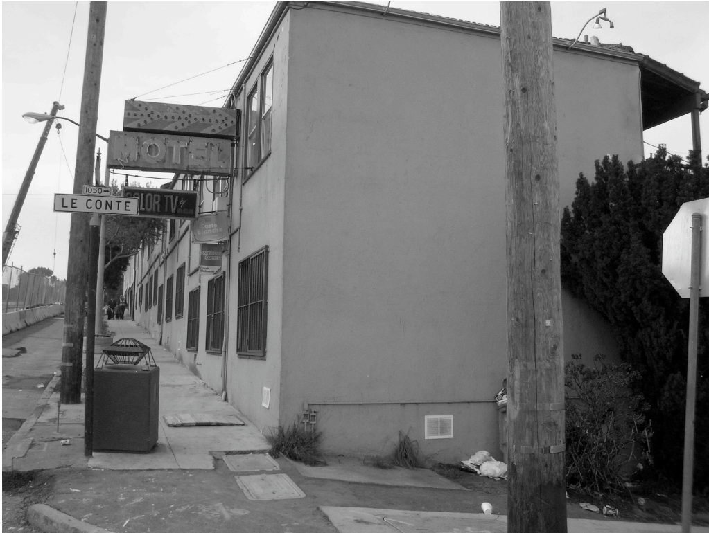
Southwest corner, Third Street and Le Conte Avenue: Extensively deteriorated motel, apparently used for long term residence. Deteriorated signage, trash accumulation, unsafe sidewalk and curb.
