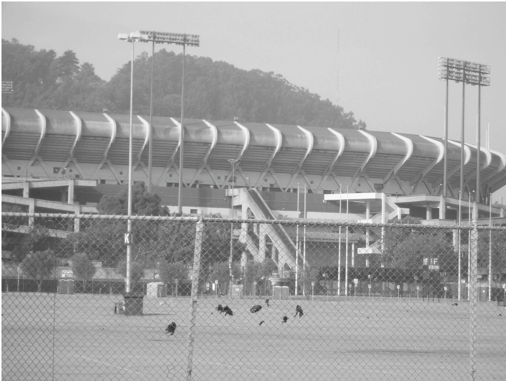
Northeast side of Candlestick Park: Deteriorated stadium, mold on upper deck, rusted light towers, cracked and uneven pavement.
