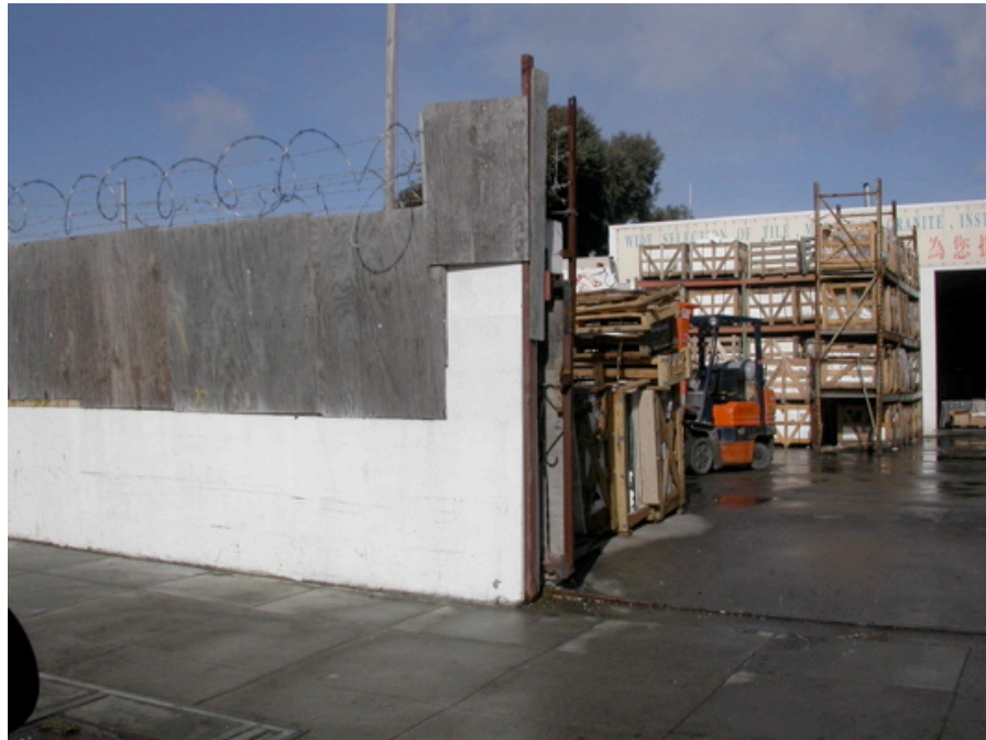
Third Street at Gilman Street: Informal construction of fence.
