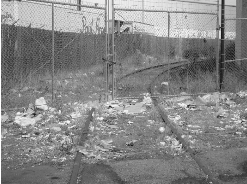
Van Dyke Avenue between Hawes and Ingalls Streets: Defunct, inoperable railroad tracks, trash accumulation.
