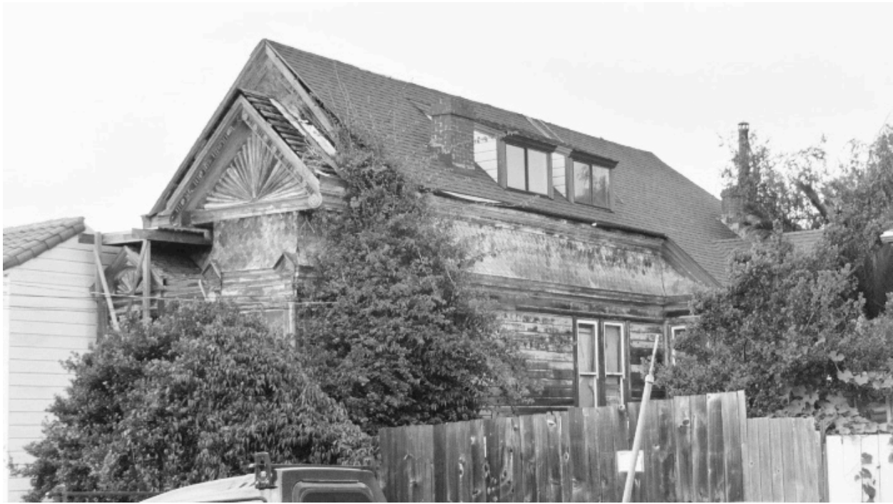
1552 Palou Avenue: Dilapidated residence, deteriorated siding and trim, peeling, chipped and fading paint, deteriorated and missing roofing materials, water damage, unreinforced masonry chimney, poorly maintained landscaping, missing gutters and downspouts.
