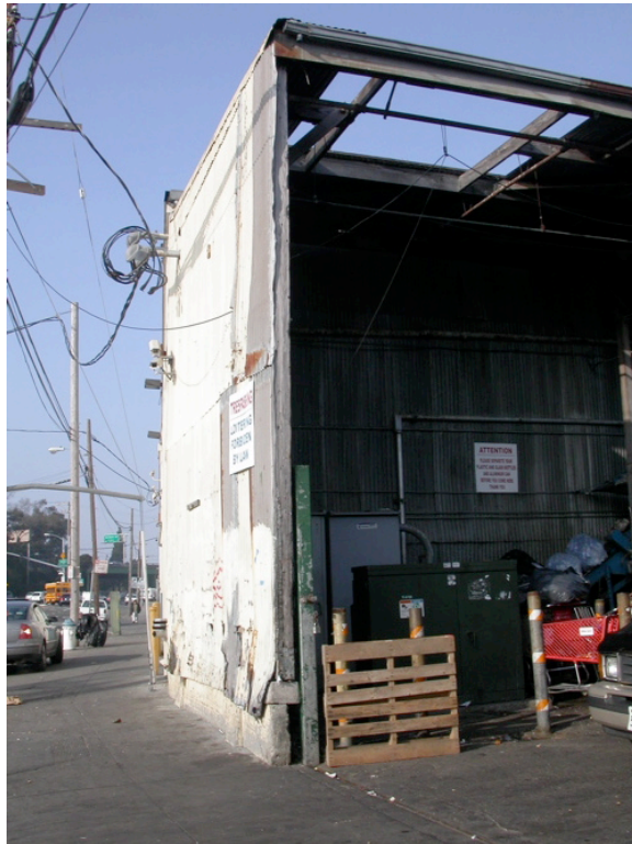
2380 Jerrold Avenue: Deteriorated, rusted corrugated steel building, graffiti on siding, lacks proper roofing, deteriorated painting.
