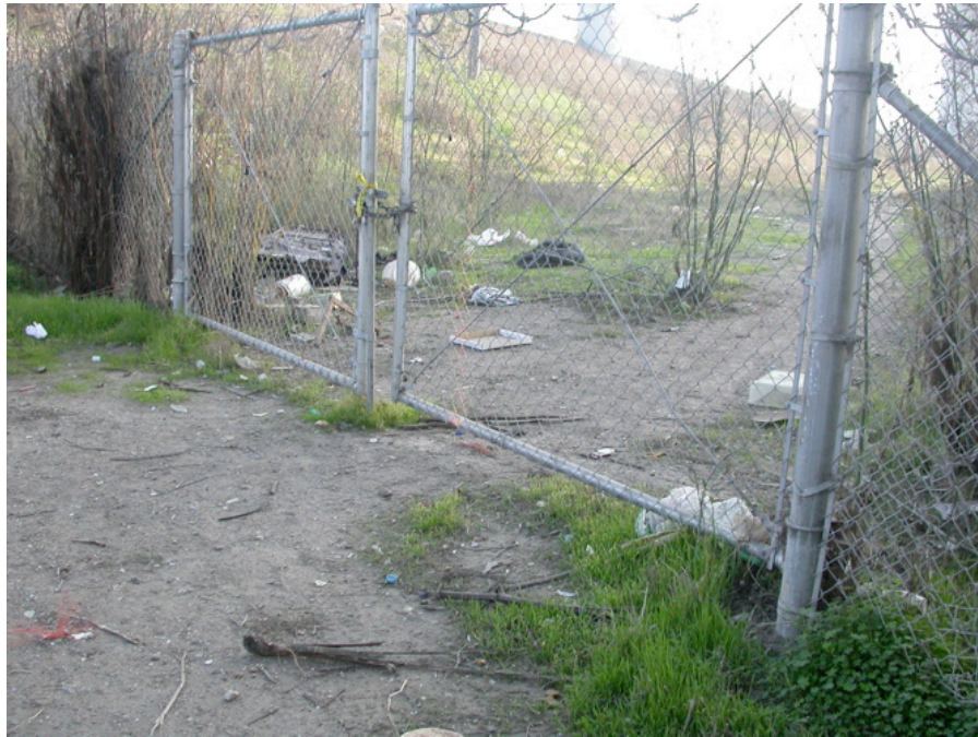
Northeast corner of Evans Avenue and Selby Street: Missing sidewalk, accumulated trash, and overgrown landscaping.
