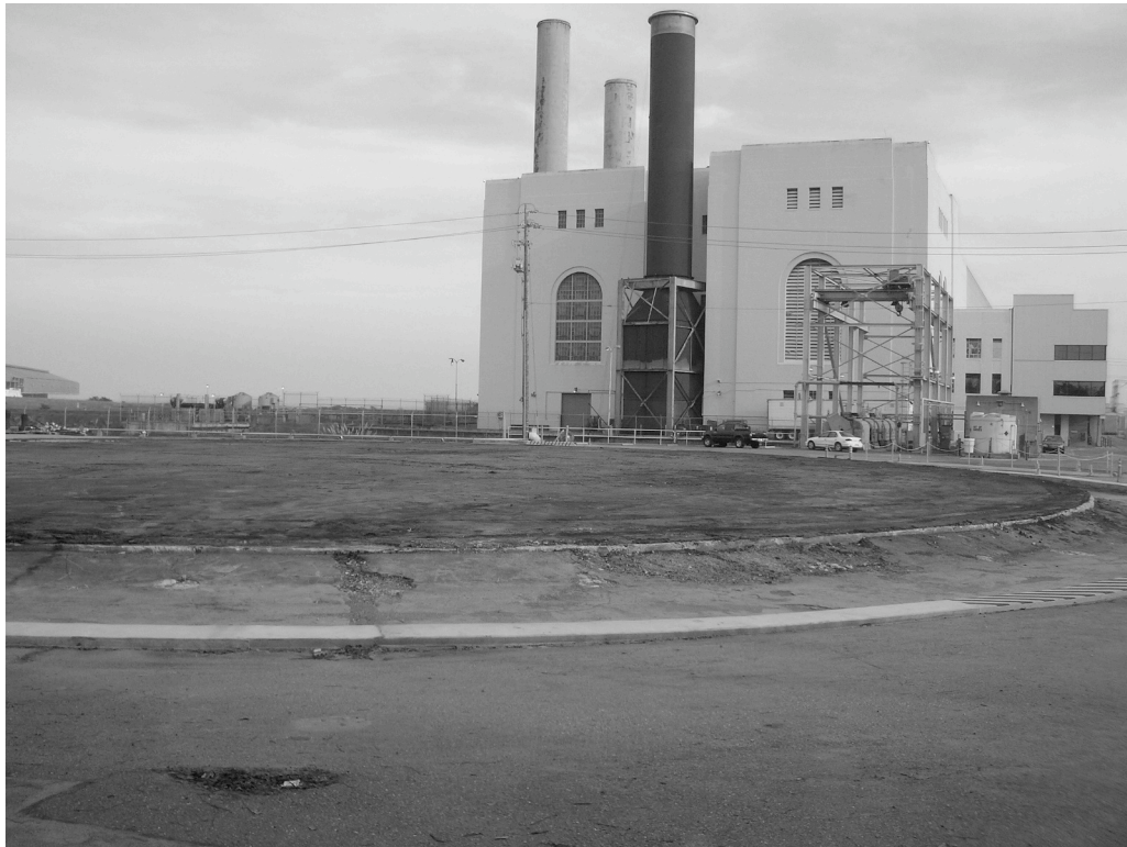
100 Evans: Site of former PG&E storage tank. Area of potential contamination.
