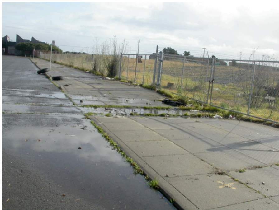
Southside of Thomas Avenue between Hawes Street and Griffith Street: Inoperable railroad tracks, and vacant and underutilized lot, standing water, and illegal tire dumping.
