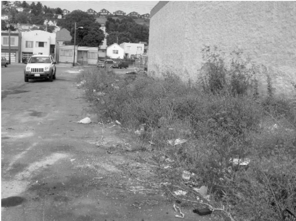
Northeast corner, Crisp Road and Revere Avenue: Lack of sidewalk, trash accumulation, deteriorated pavement, poorly maintained landscaping.
