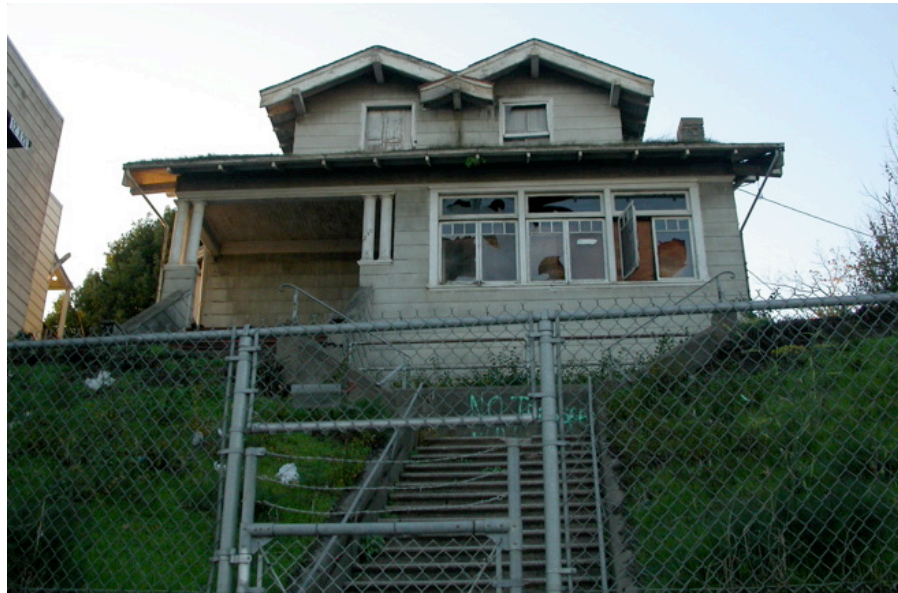
5250 3 rd Street: Vacant dilapidated residence, broken windows, boarded windows, missing gutters and downspouts, deferred maintenance, overgrown landscaping.
