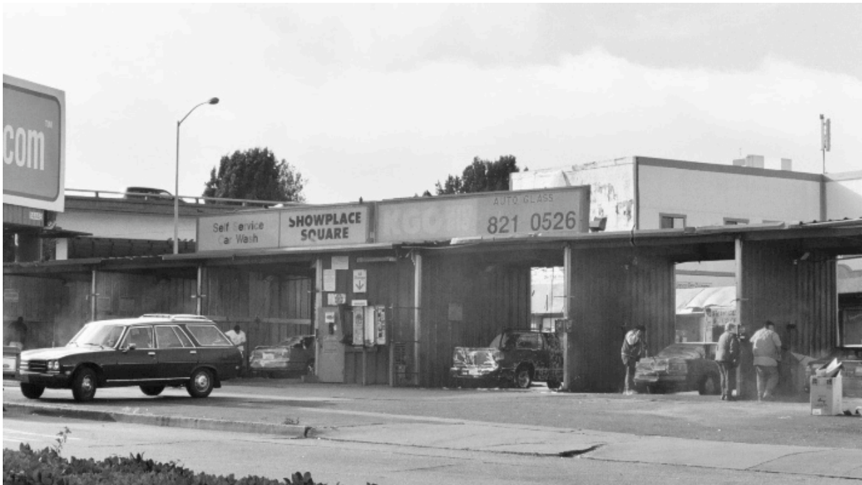
Northeast corner, Marin Street and Bayshore Boulevard: Extensively deteriorated structure, alignment problems, deteriorated signage, sagging and deteriorated roof, missing gutters; deteriorating pavement.
