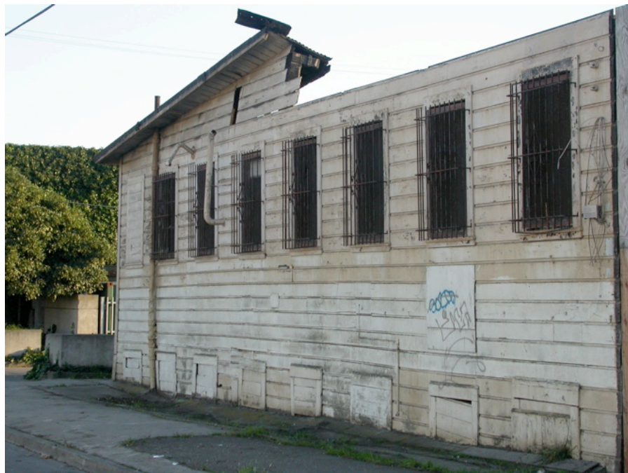
Southwest corner, Thomas Avenue and Hawes Street: Remaining shell of vacant, fire damaged residence, substandard construction, deteriorated painting, incomplete siding, missing gutters, graffiti, and cracked sidewalk.
