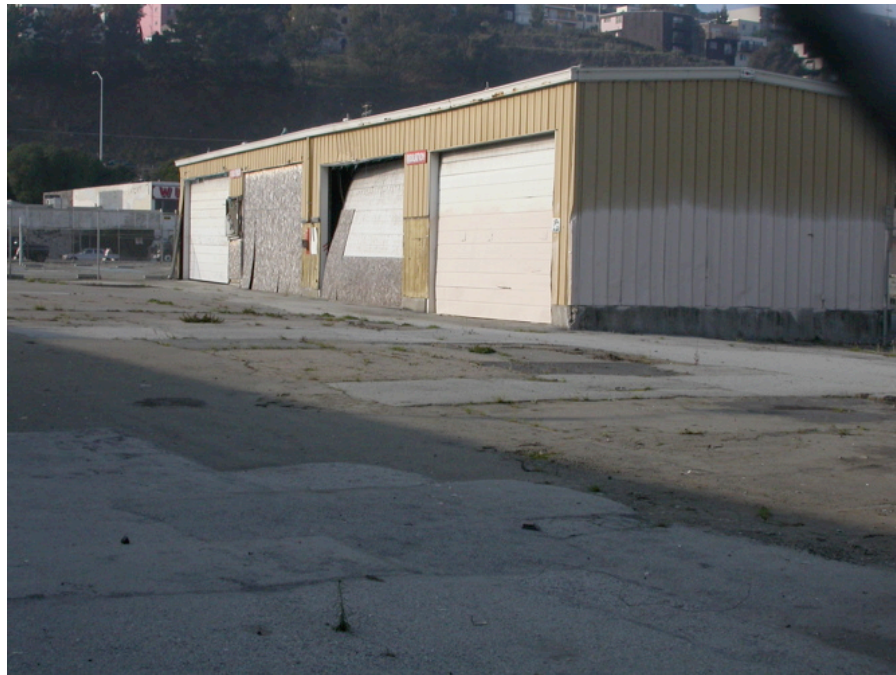
East side of Bayshore Boulevard at Cortland Avenue: Extensively deteriorated vacant structure on site of former Goodman's Lumber, deteriorated and warped siding, boarded doors, deteriorated gutters.
