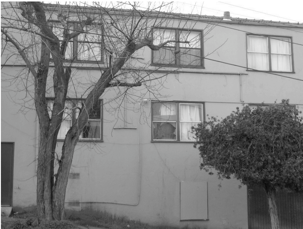
Southwest corner, Third Street and Le Conte Avenue: Extensively deteriorated motel. [Detail of building above]
