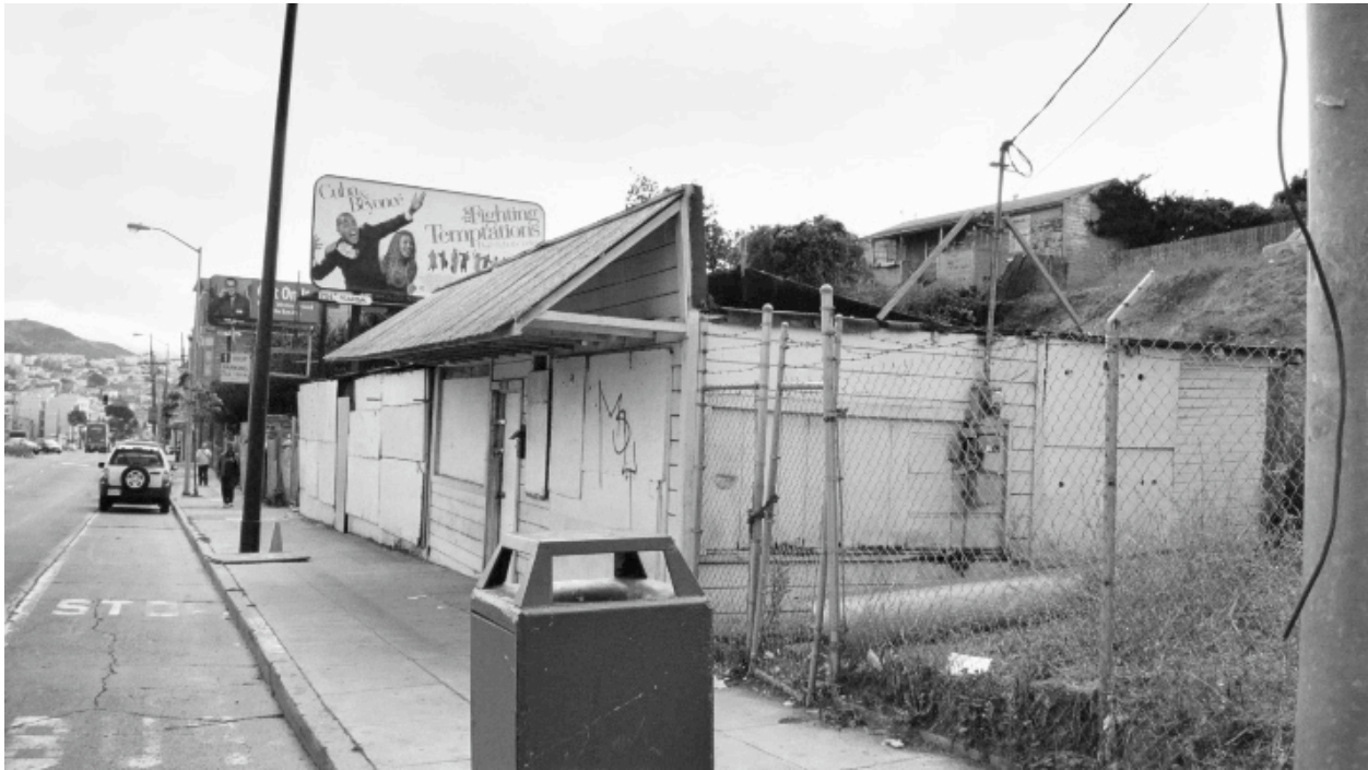
5210-16 Third Street: Dilapidated structure, deteriorated and sagging walls, roof and overhang deferred maintenance, deteriorated paint, boarded windows, missing gutters and downspouts.
