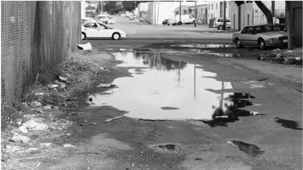
Newcomb Avenue, between Selby and Toland Streets: Large areas of standing water, deteriorated pavement, lack of sidewalks, accumulated debris.
