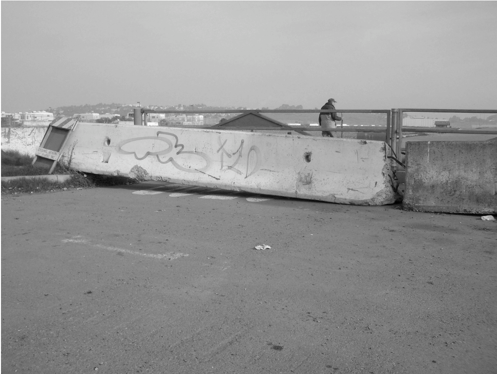
Donahue Street at Gilman Avenue, towards the northeast: Underutilized lot. Deteriorated barriers.
