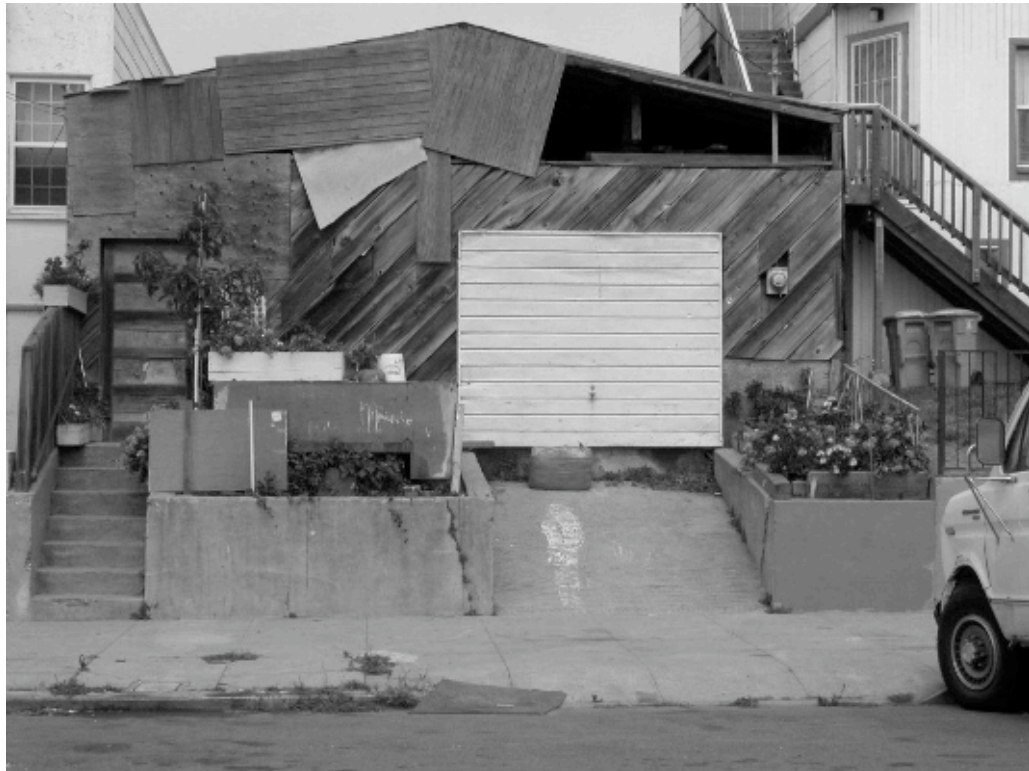
1218 Egbert Avenue: Dilapidated building, informal and substandard construction, deferred maintenance, large hole in front façade, deteriorated siding, large cracks in retaining wall, deteriorated sidewalk.
