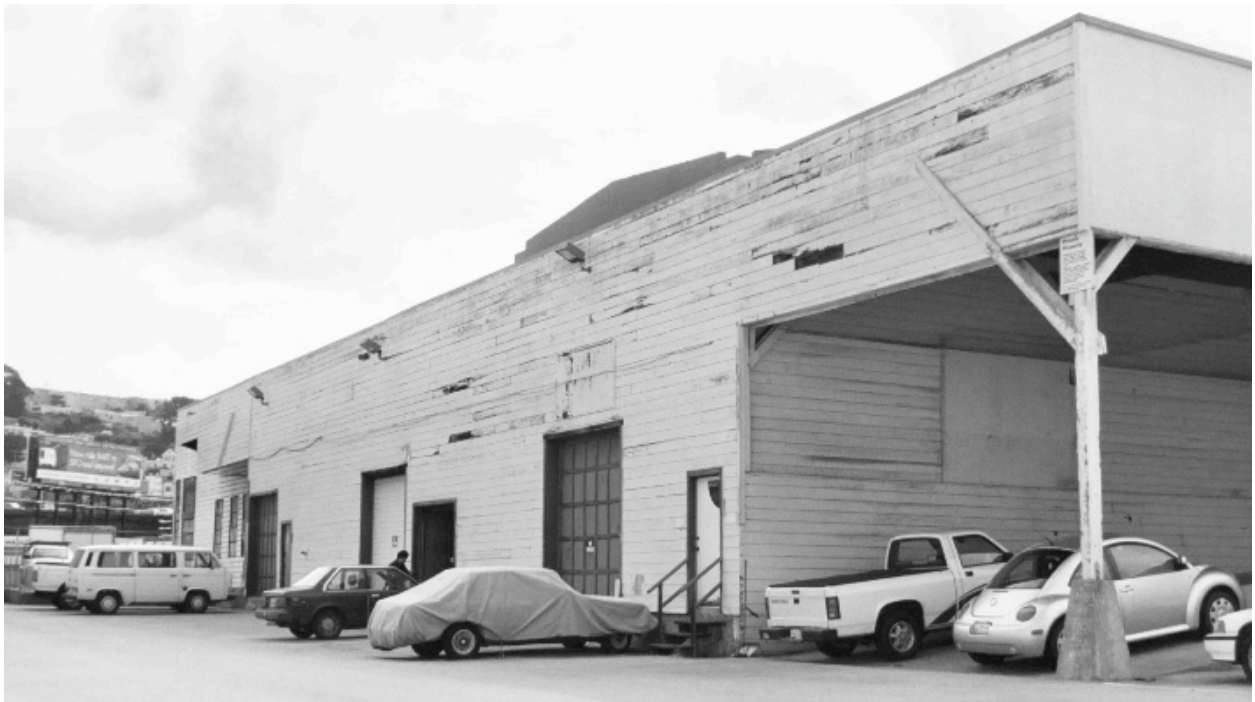
1485 Bayshore Blvd (Rear): Extensively deteriorated building, deferred maintenance, holes in wood siding, deteriorated paint, mold and water damage.
