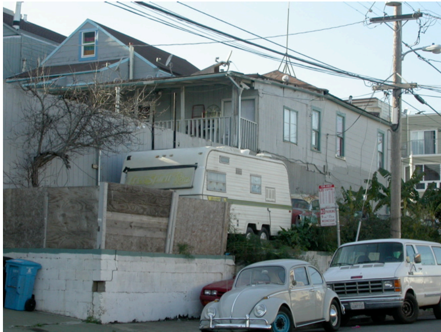
2901 Hawes Street: Inoperable vehicles, deteriorated siding, cracks in concrete retaining wall, informal and substandard construction, deteriorated gutters.
