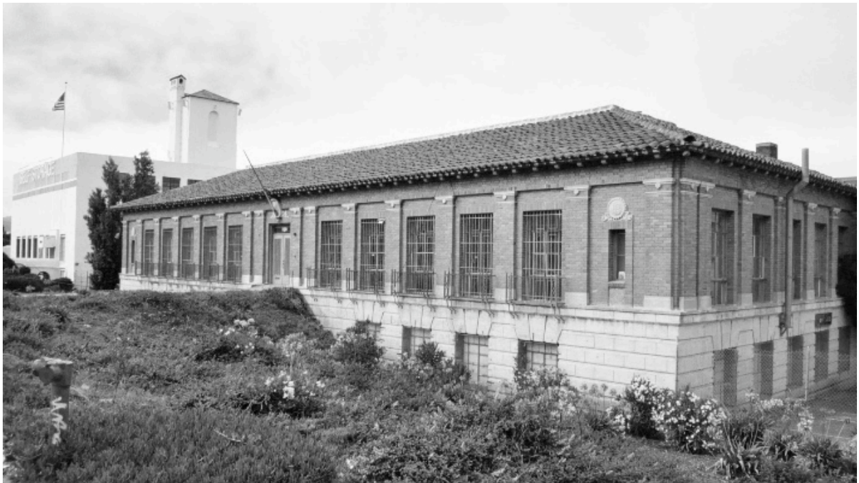
320 Paul Avenue: Vacant, unreinforced masonry building, cracks in concrete, deteriorating roof.
