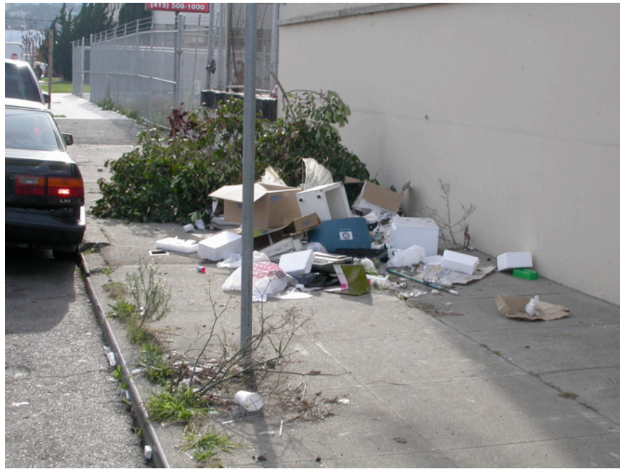
2626 Newhall Street at end of Lydia Street: Trash accumulation, deteriorated sidewalks, overgrown landscaping encroaching on sidewalk.
