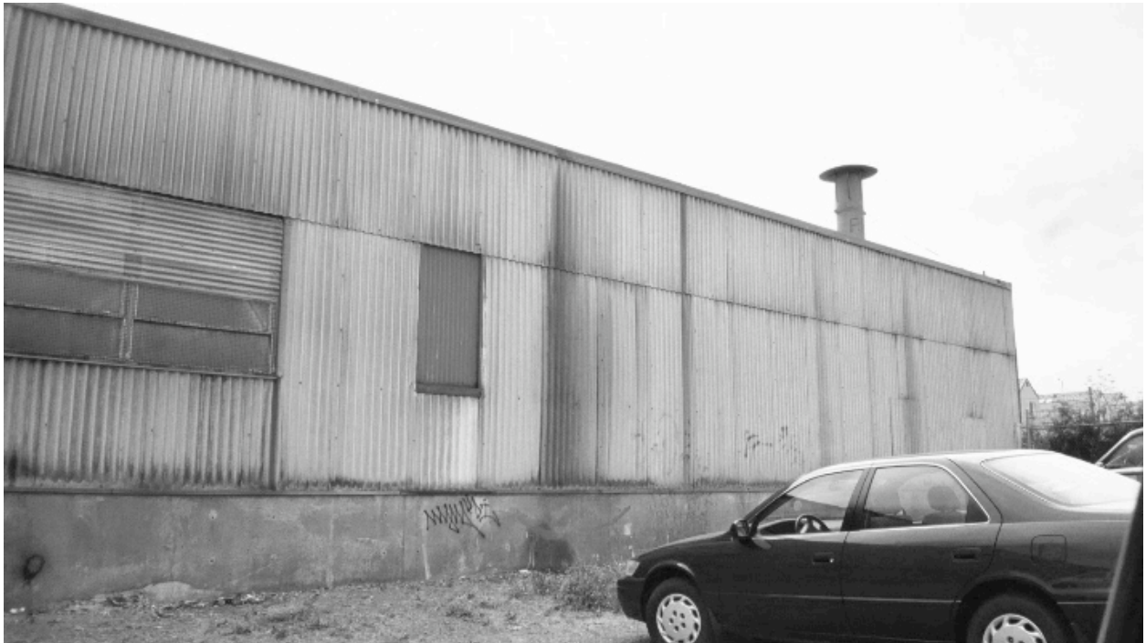
South side of Armstrong Avenue between Mendell and Third Streets: Dilapidated building, extensively deteriorated, sagging and rusted siding, lack of sidewalk, graffiti.
