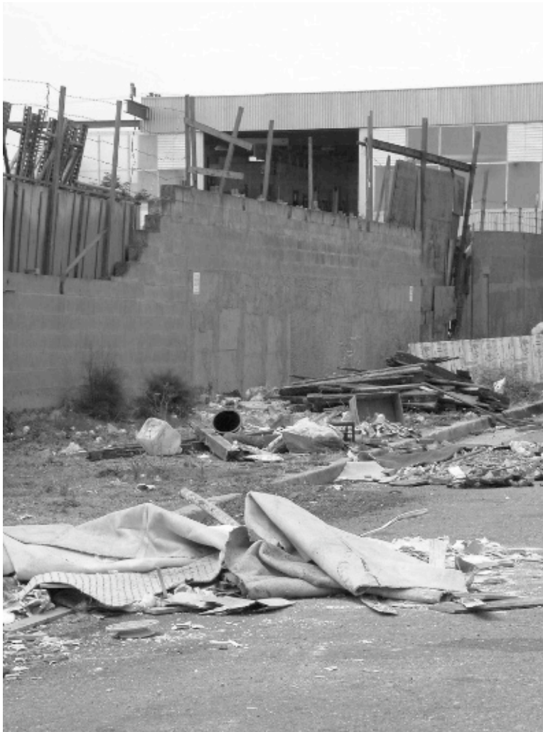
Southeast corner, Van Dyke Avenue and Hawes Street: Significant trash accumulation, illegal dumping, partially constructed and deteriorated wall.
