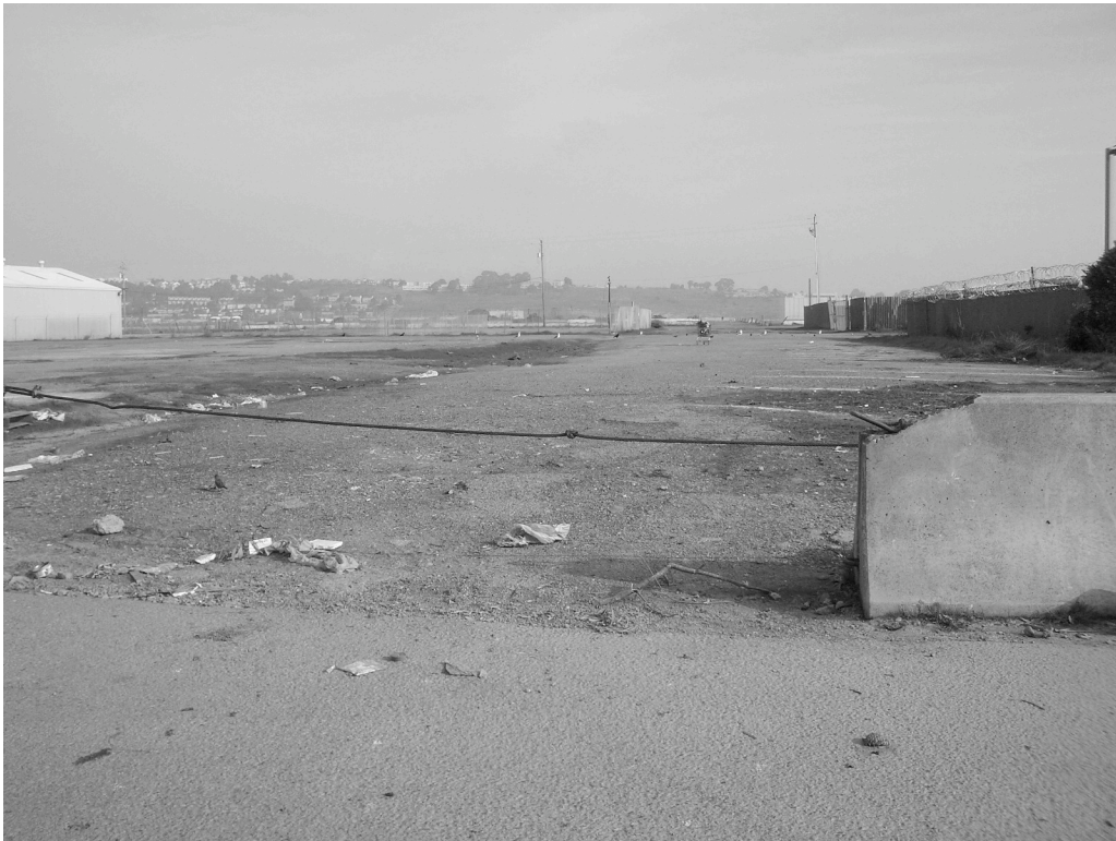
Earl Street at Gilman Avenue, toward the northeast: Unpaved public street and unpaved parking lot used for 49ers games at Candlestick Park. Deteriorated barrier, trash accumulation.
