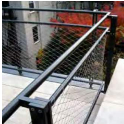
Stainless Steel Cable Mesh Guardrail (See Page 61)
