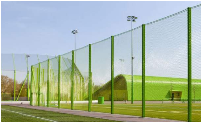
(R6) Multi-Sport Court Fence and Gate 1" PVC coated chainlink (custom color), painted support bars, rounded corners per plan
