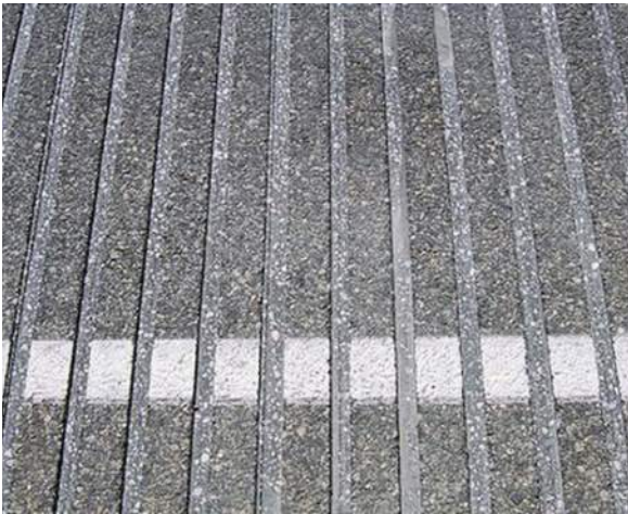
P10 Bike Rumble Strip Texturized CIP concrete
