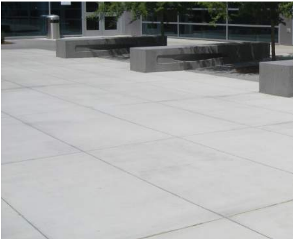
P1 CIP Concrete Natural gray with sawcut joints 3' on center each way
