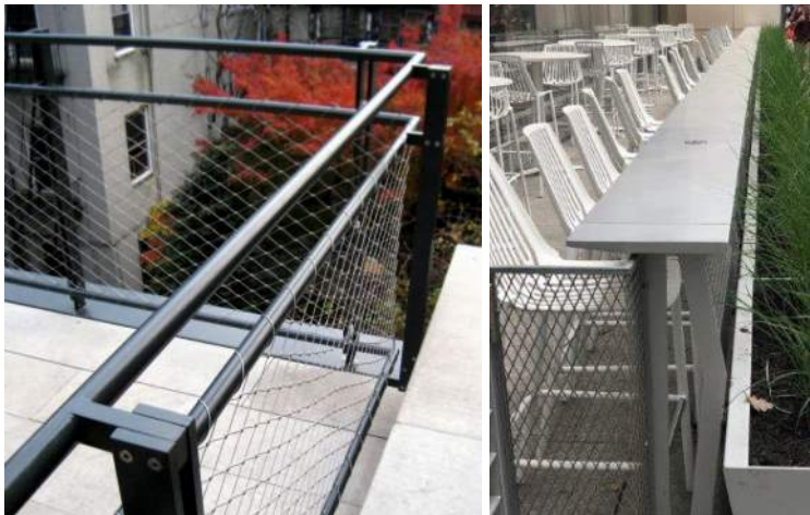
(R5) Guardrail/Bar Rail/Counter Custom painted steel rail and bar counter space with inset stainless steel mesh panels - Jakob Rope Systems "Webnet" or similar
