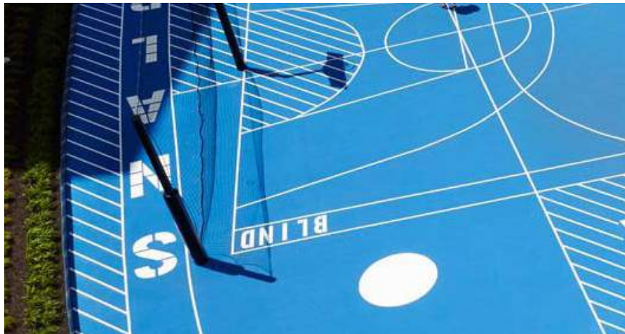
(P17) Multi-Sport Court Acrylotex Plexicourt in graphic pattern. CIP concrete float.
