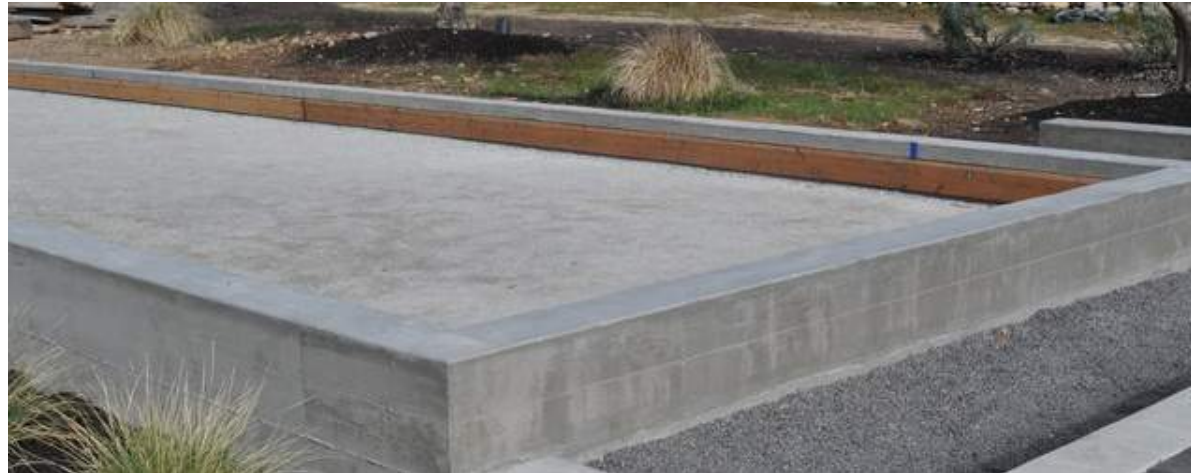
F4 Bocce Court CIP concrete curb wall with decomposed granite with oyster shell court, accessible
