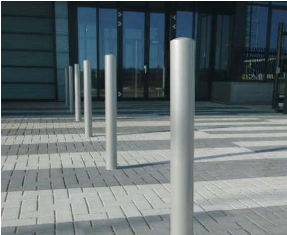
F1 Bollard Calpipe Security Bollards: 3" dia. x 42" tall, galvanized steel, embed mount, removable as needed
