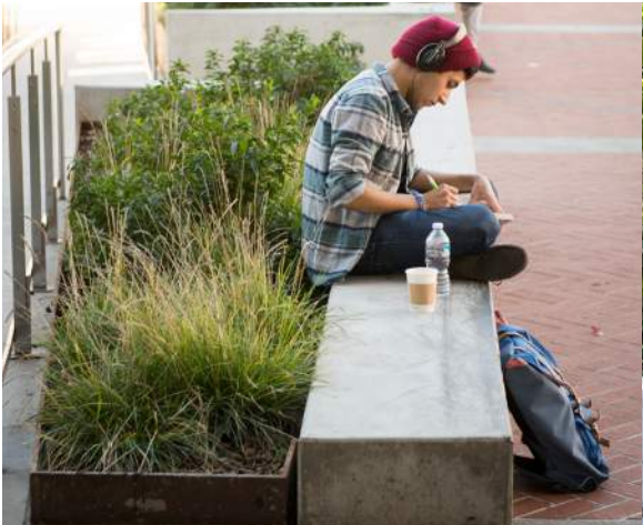
(S4) Seatwall Precast/architectural finish concrete. With/without backrest
