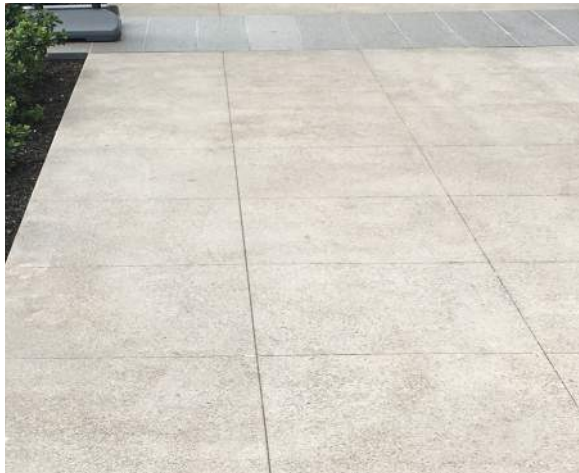
P4 CIP Concrete Integral color 'Sandstone' sawcut joints 4' on center each way (to match Folsom)
