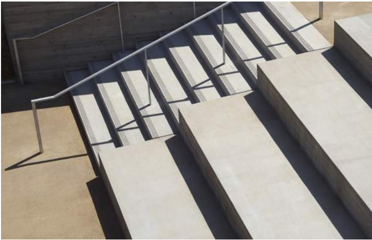
(S5) Lawn Terrace Precast/architectural finish concrete with inset synthetic lawn panels
