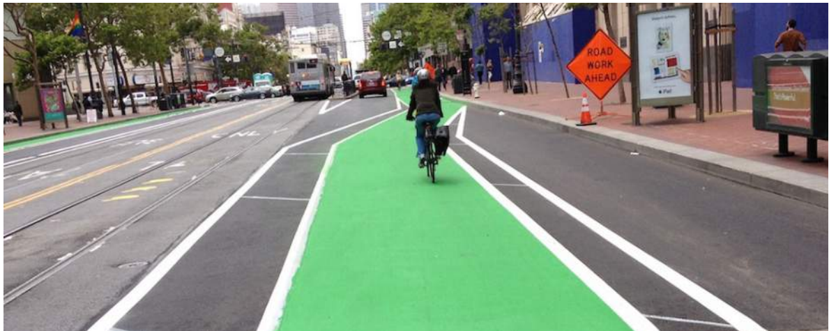
P8 Bike Lane Asphalt with thermoplastic paint
