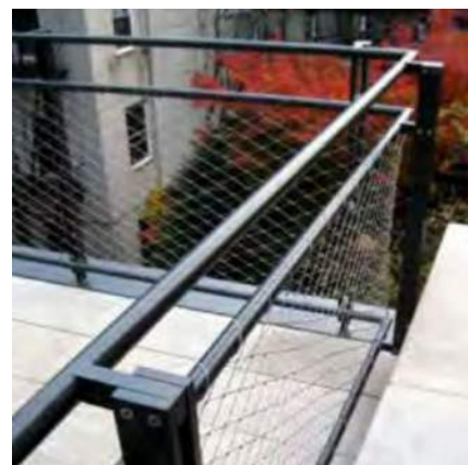
Stainless Steel Cable Mesh Guardrail (See Page 61)
