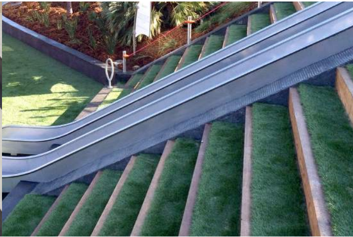
(S5) Lawn Terrace Precast/architectural finish concrete with inset synthetic lawn panels
