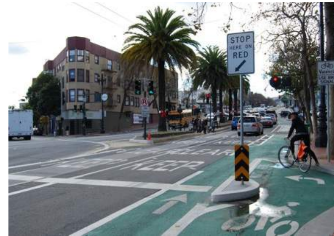
(P19) Pedestrian and Bicycle Striping Thermoplastic on asphalt roadway
