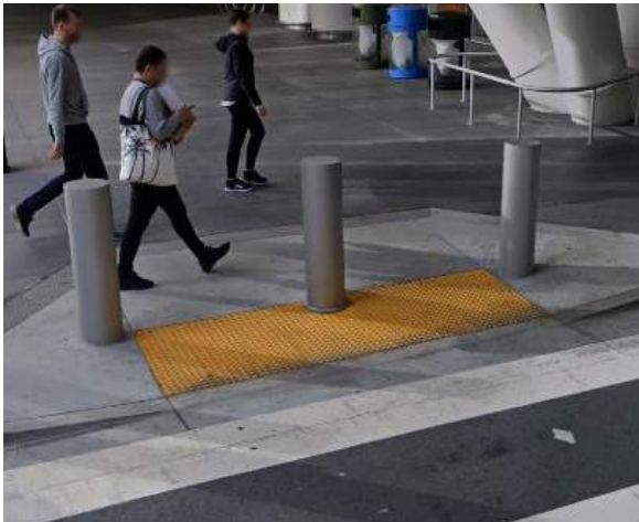
P3 Detectable Warning Precast concrete Pavers
