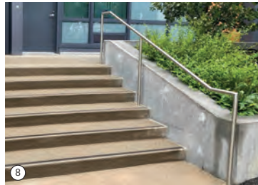
8 Stairs At Stoops
