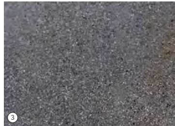
3 Integral Color Concrete Banding
