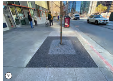
9 Porous Gravel Paving
