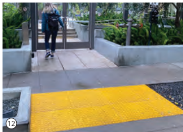
12 Truncated Domes at Raised Crossings
