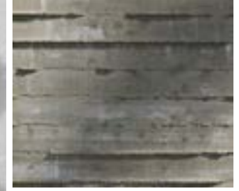
2 Board form Concrete Planter Wall
