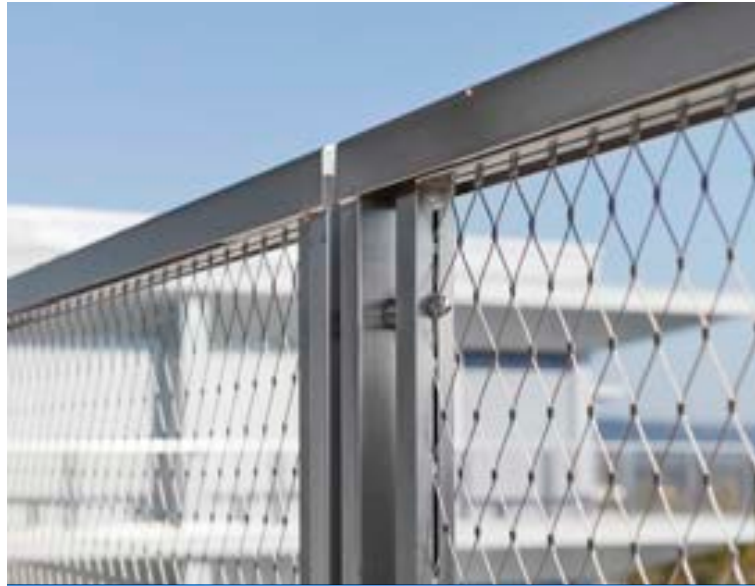
Roof Railings: Metal and Cable Net
