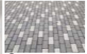
1 6"X12" Concrete Unit Pavers In Two Colors With Ground Face Finish In Stacked Bond With Linear
