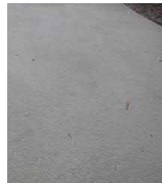
Crushed Stone Surfacing
