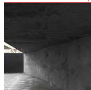
8 Grand Entry Canopy: Precast Concrete
