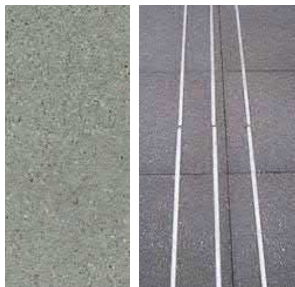
Poured in Place Concrete Paving w/ metal strip inlay
