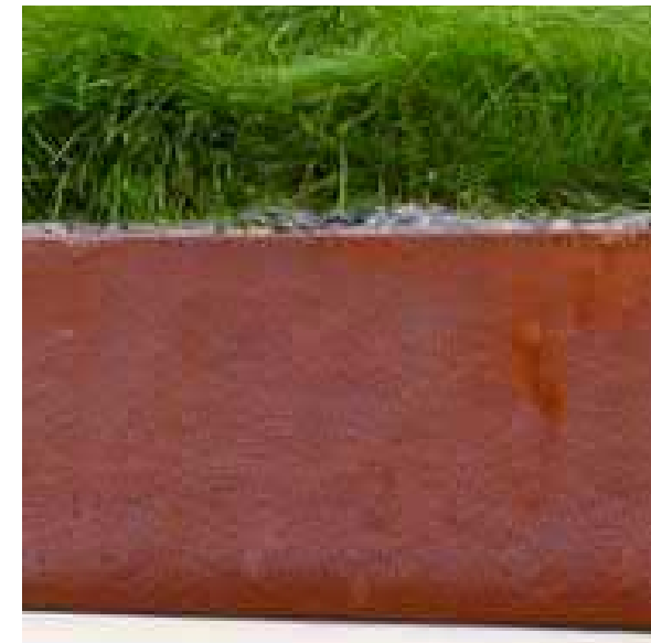
Weathered Steel edging
