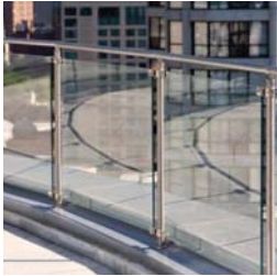
1 42" HT. EXTERIOR ALUM. TEMPERED GLASS RAIL
