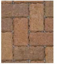
2 PERMEABLE PAVERS INTERLOCKING BLOCK PAVERS
