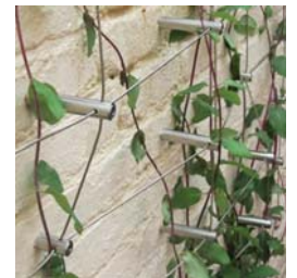
10 GREENWALL CABLE SYSTEM, TYP.
