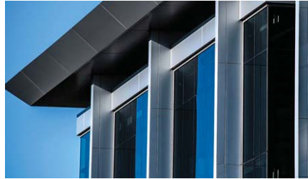
3 ALUMINUM RAINSCREEN SYSTEM BY ALUMAWALL "1800 SERIES", OR EQ
