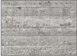
7 WOOD GRAIN CONCRETE WALL
