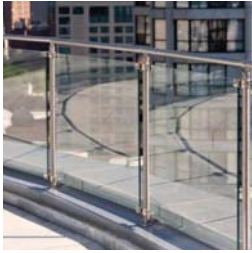
1 42" HT. EXTERIOR ALUM. TEMPERED GLASS RAIL
