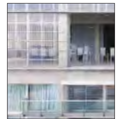
GLASS Façade/ CONCRETED STRUCTURE
