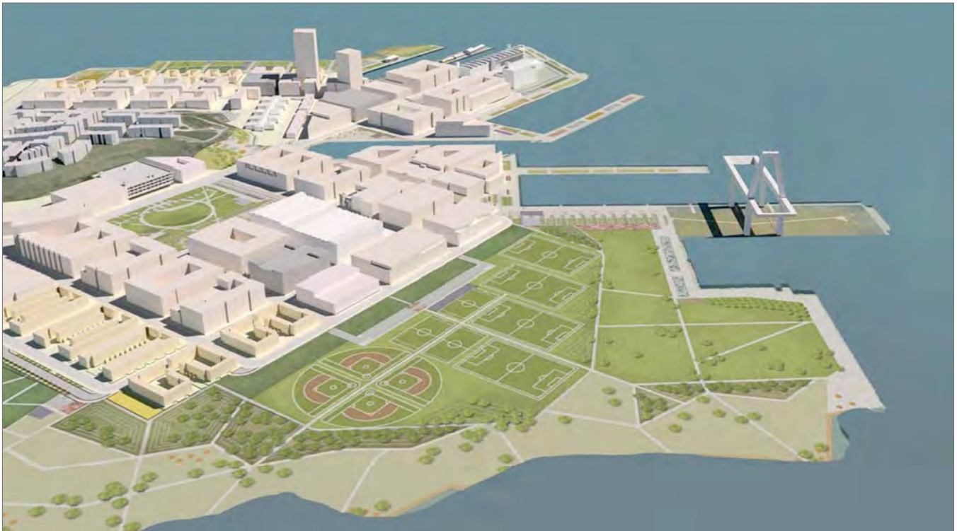
Figure 4.2d: VIEW LOOKING NORTH
