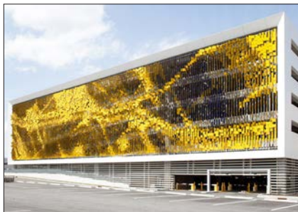
Precedent: Example of enhanced screening at Eskenazi Hospital Parking Garage. Credits: Serge Hoeltschi, https://www.architectmagazine.com/technology/detail/detail-mayseptember-installation-at-eskenazi-hospital-parking-garage_o , https://www.rob-ley.com/may-september .
