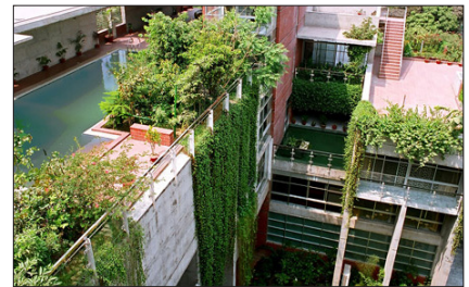
Precedent – Façade articulation.
