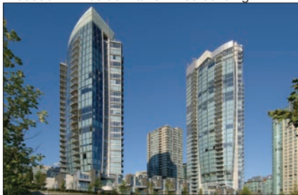
Precedent – Residential high-rise building.
