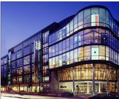
Precedent – Commercial at corner.
