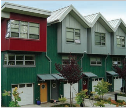
Precedent – Garage entrance off private driveway.
