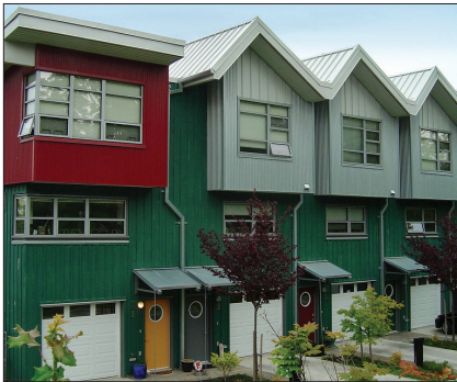
Precedent – Townhome garage entrance.
