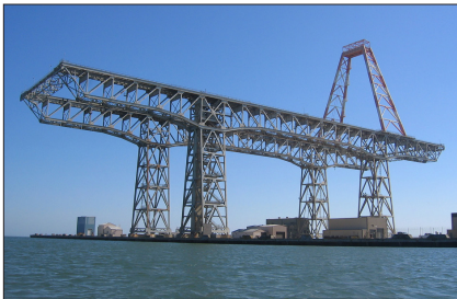
Landmark – Shipyard crane.
