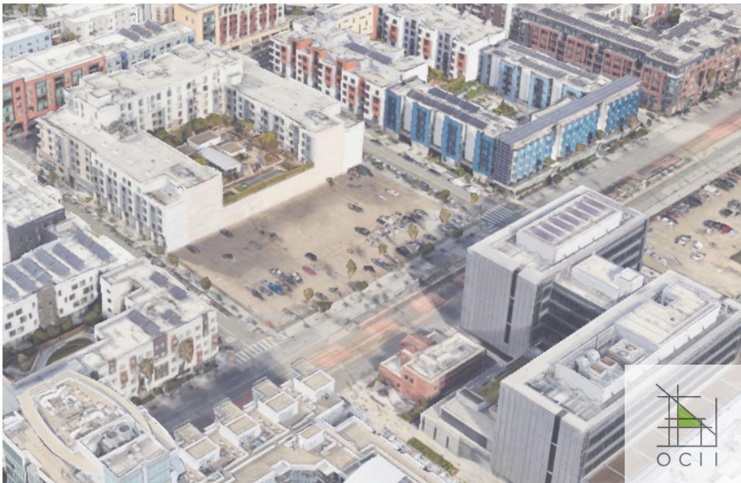
View of Mission Bay South Block 4 East from Third and China Basin Streets looking northwest
