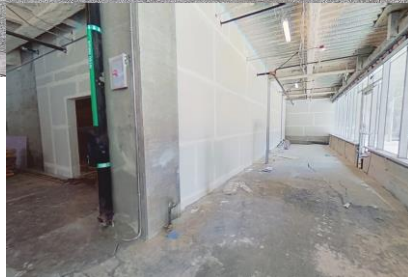
PHOTO EXISTING CONDITIONS TMM MAIN ENTRANCE PROPOSED WALL WRAP BANNER
