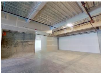
PHOTO EXISTING CONDITIONS
