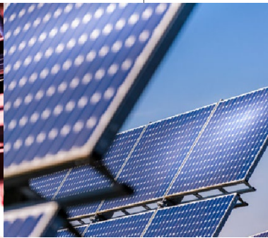
Solar Energy & Battery Storage
