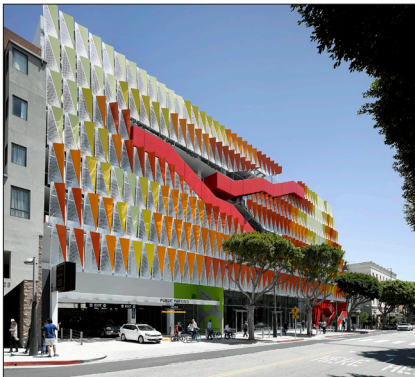
Precedent: Example of enhanced screening using graphic facades. Credits: CoSM Public Parking Structure, Behnisch Architekten with Studio Jantzen and IPD, Photo © David Matthiessen.
