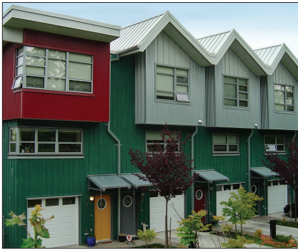
Precedent – Townhome garage entrance.
