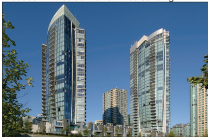
Precedent – Residential high-rise building.
