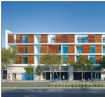
Precedent – Facade Variation with change in material , color, and texture. Credits: Koning Eizenberg Architecture, Photo © Eric Staudenmaier.
