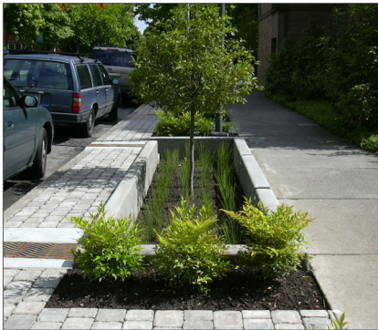
Precedent – Bioswale storm water garden.
