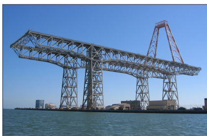
Landmark – Shipyard crane.
