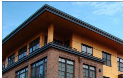
Precedent – Distinctive roof.
