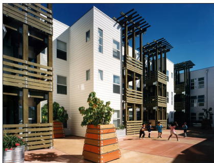
Precedent – Internal courtyard.
