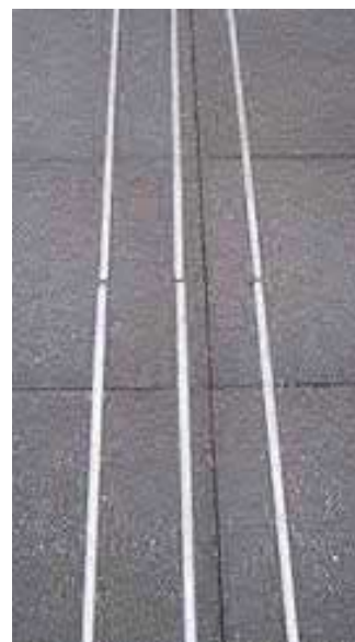
Poured in Place Concrete Paving w/ metal strip inlay
