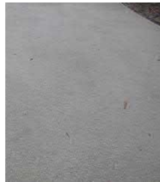
Crushed Stone Surfacing
