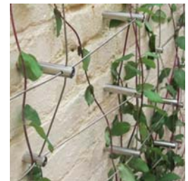
⑩ GREENWALL CABLE SYSTEM, TYP.
