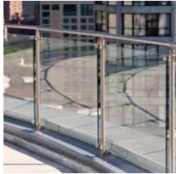
① 42" HT. EXTERIOR ALUM. TEMPERED GLASS RAIL
