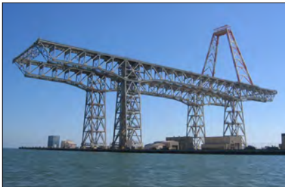
Landmark – Shipyard crane.
