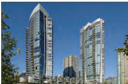
Precedent – Residential high-rise building.
