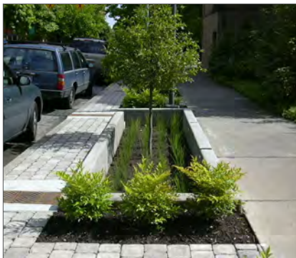
Precedent – Bioswale storm water garden.
