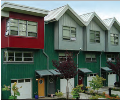
Precedent – Townhome garage entrance.
