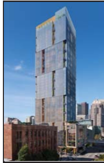
Block 9 500 Folsom St. Developers: Essex/ BRIDGE Affordable Rental Units: 109 AMI: 50% & below Market-Rate Rental Units: 428 Total Units: 537 Construction Start: 2016 Completion: 2020
