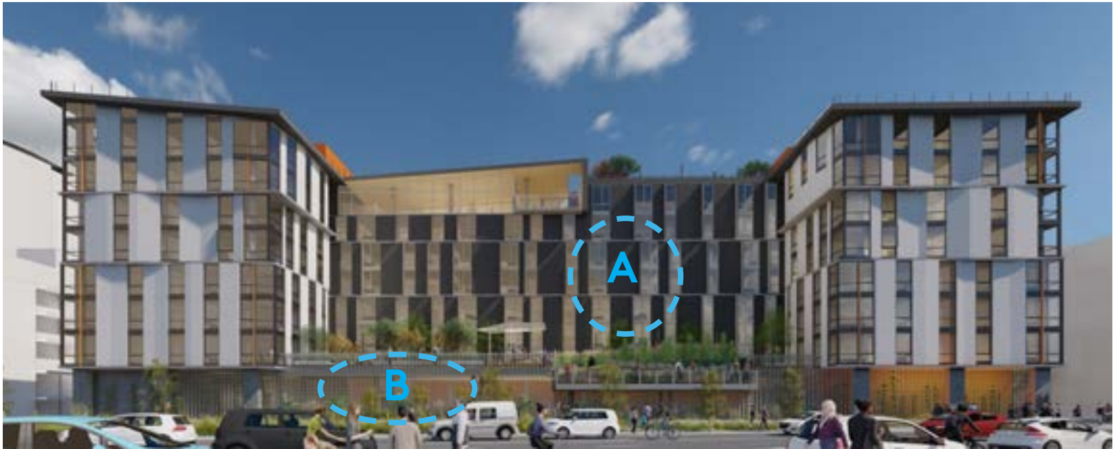
B. ALUMINUM PERFORATED PANELS, DIFFERING PERFORATIONS AT GARGE AND TERRACE
