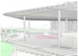
4 BOK Modern Steel Trellis Structure
