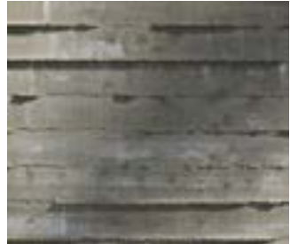
2 Board form Concrete Planter Wall
