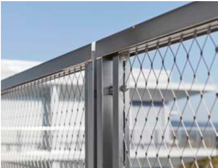
Roof Railings: Metal and Cable Net
