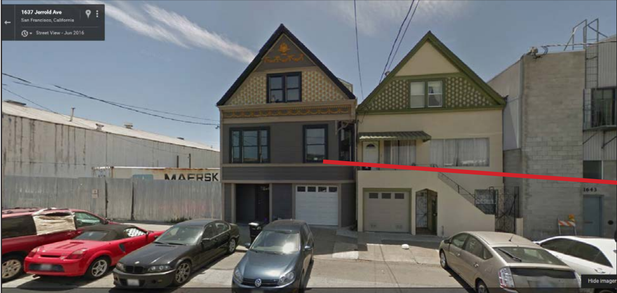
JERROLD AVE, NORTHWEST NEIGHBORING PROPERTIES
