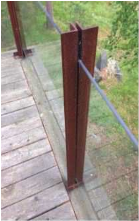
TEMPERED GLASS AND CORTEN ANGLE BALCONY RAILING
