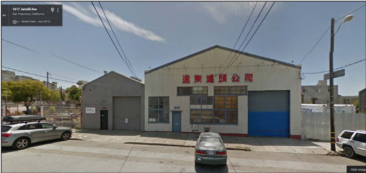
JERROLD AVE, SOUTHEAST NEIGHBORING PROPERTIES
