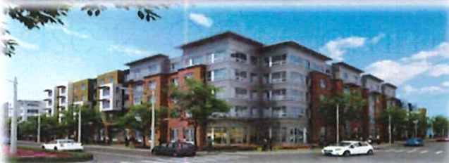
Alice Griffith Phase 3 Block 1 122 units SF Housing Development Corp.
