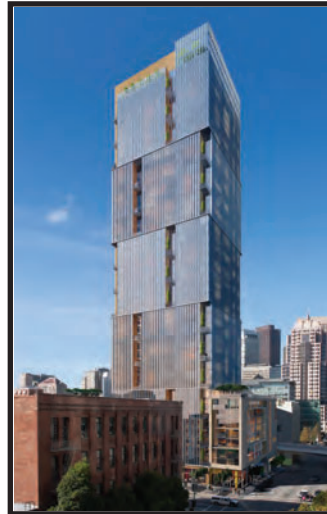
Block 9 500 Folsom St. Developers: Essex/ BRIDGE Affordable Rental Units: 109 AMI: 50% & below Market-Rate Rental Units: 436 Total Units: 545 Construction Start: 2016 Completion: 2019
