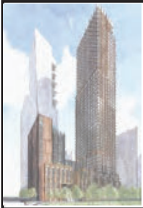
Block 4 Developer: Hines/Urban Pacific/ Goldman Sachs Affordable Rental Units: 336 AMI: 45% - 100% Market-Rate Rental & Condo Units: 347 Construction Start: 2021 Completion: 2024
