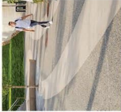
CONCRETE BANDING INTEGRAL COLOR WITH BROOM FINISH
