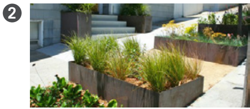
RAISED STEEL FLOW-THROUGH STORM WATER
