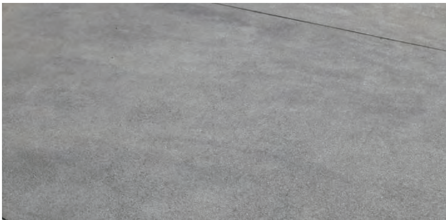
4 INTEGRAL COLOR CONCRETE PAVING COLOR: GRAPHITE
