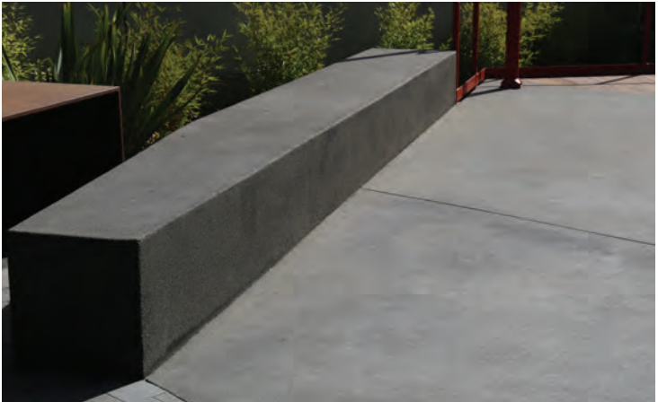
6 INTEGRAL COLOR CONCRETE WALL COLOR: GRAPHITE
