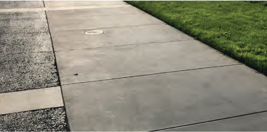
2 EXISTING CONCRETE HARDSCAPE TO REMAIN
