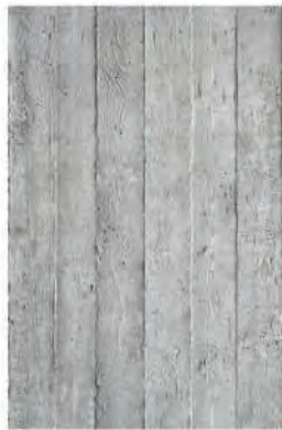
B AT-GRADE EXTERIOR: VERTICAL BOARD FORMED CONCRETE
