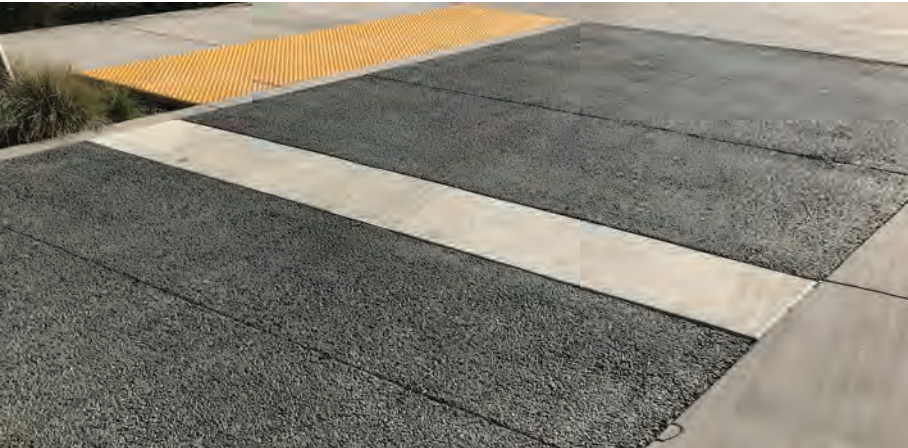
4 EXISTING CONCRETE ACCENT BANDS
