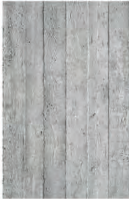
B AT-GRADE EXTERIOR: VERTICAL BOARD FORMED CONCRETE
