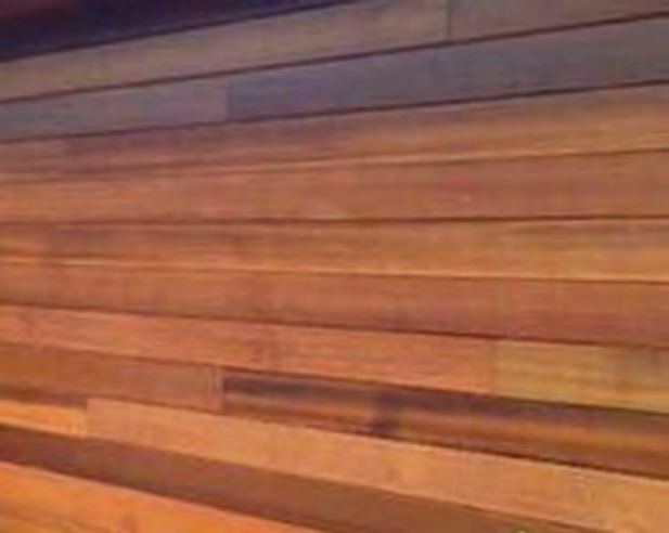
SOFFIT AT ENTRY AND COMMUNITY ROOM PERGOLA: STAINED WOOD
