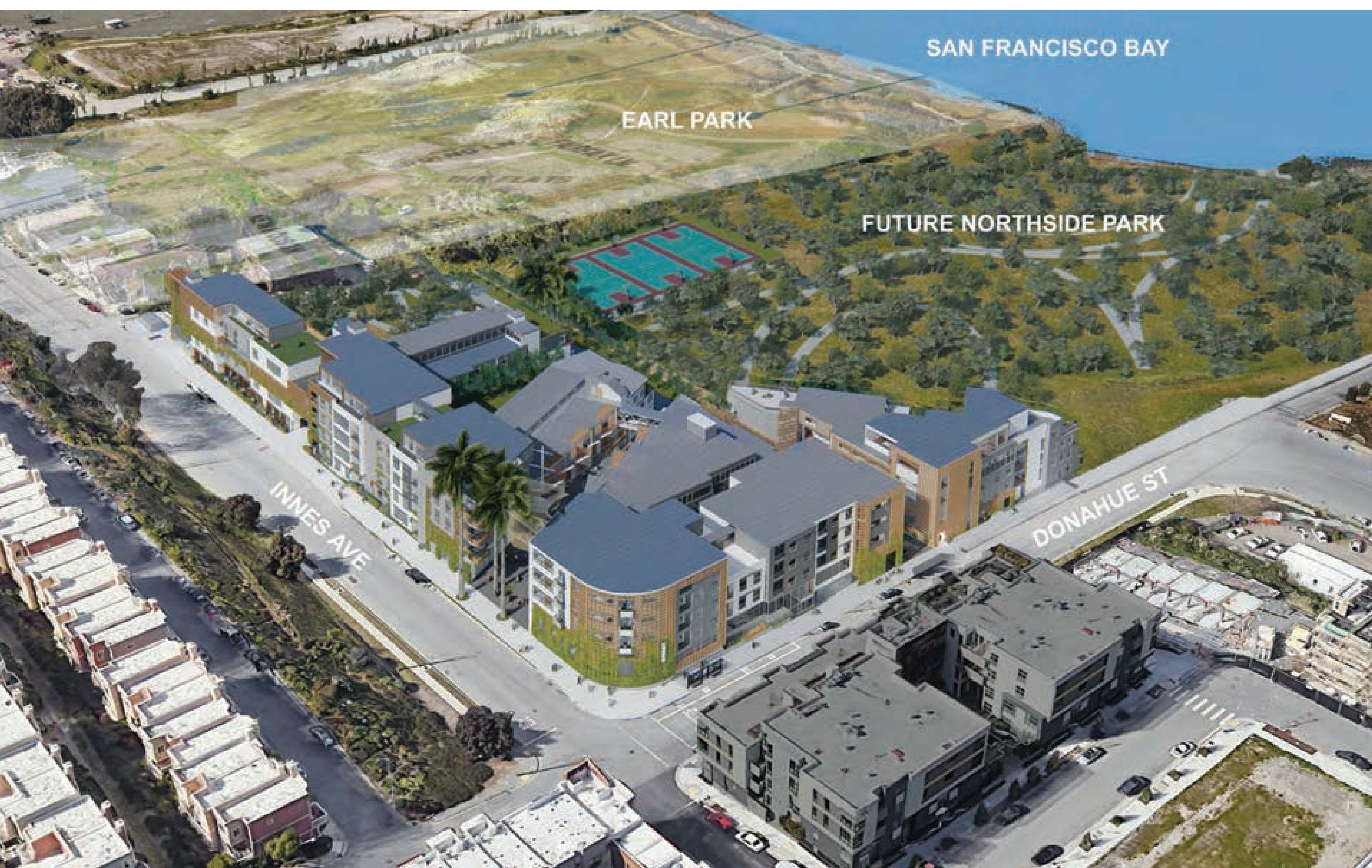
VIEW 1: AERIAL VIEW LOOKING TOWARDS THE BAY NOTE: SEE A101 FOR VIEW LOCATION
