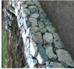
Dry Stack Stone Wall
