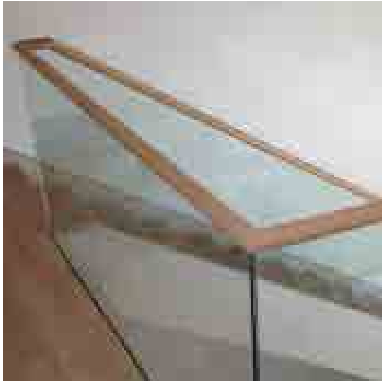
3. GLASS RAILING WITH WOOD CAP
