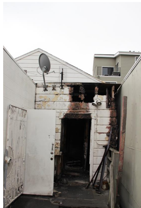
Figure 14. South part of rear façade, second floor
