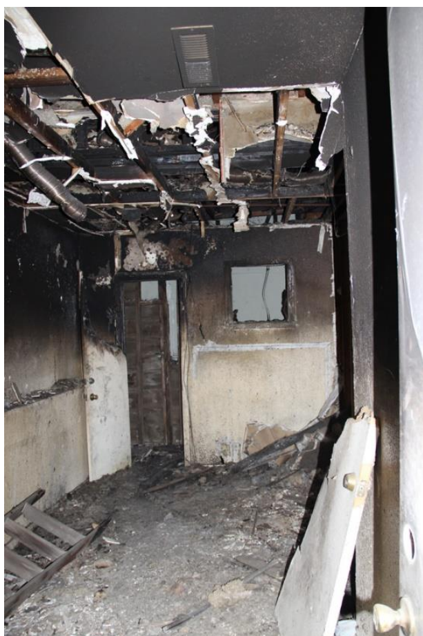
Figure 19. Second floor residential unit; view toward north
