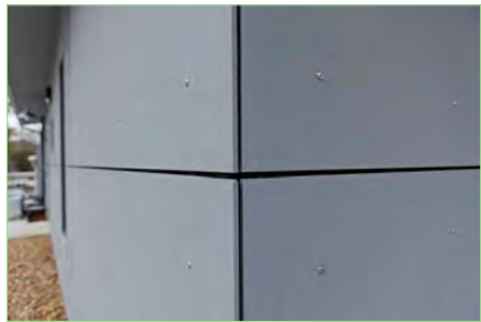
RAIN SCREEN (CORNER DETAIL)
