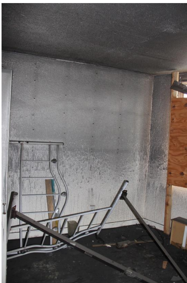
Figure 20. Second floor residential space; view toward north
