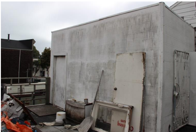
Figure 15. North part of rear façade, second floor
