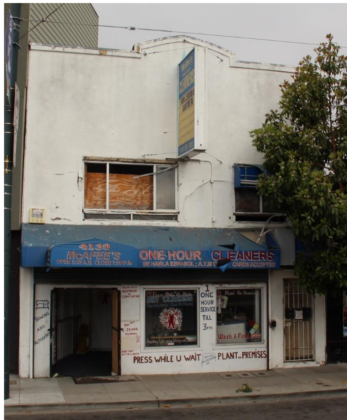
Figure 11. East (primary) façade
