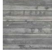
BOARD-FORMED CONCRETE MATERIAL E
