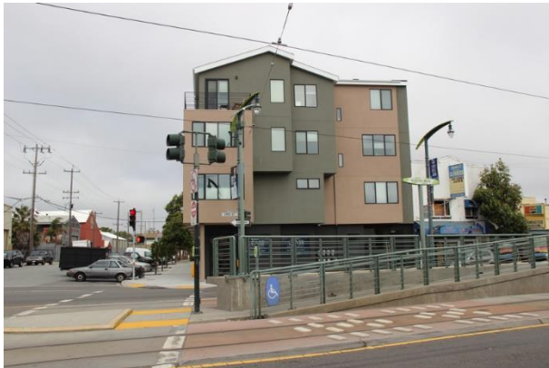
Figure 6. Condominium complex at 4132 3 rd Street; view toward west
