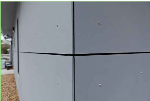
RAIN SCREEN (CORNER DETAIL)
