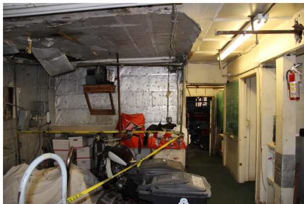
Figure 17. First floor level; view toward west
