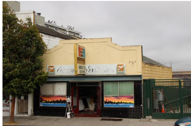
Figure 7. Constanso's Sandwich Shop, 4124 3 rd Street; view toward west
