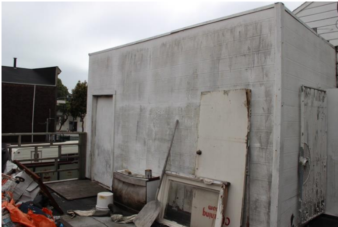
Figure 15. North part of rear façade, second floor
