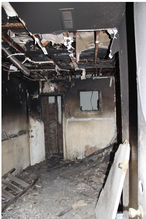
Figure 19. Second floor residential unit; view toward north
