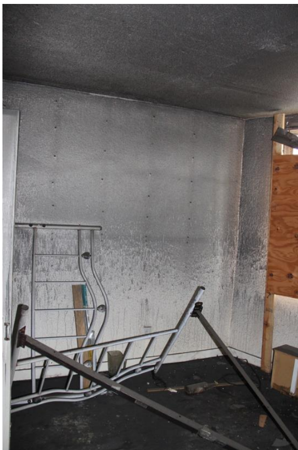
Figure 20. Second floor residential space; view toward north
