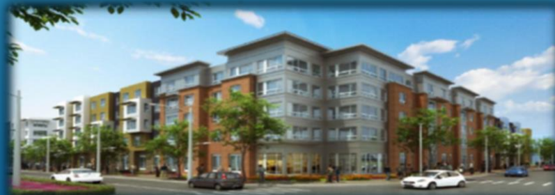
Alice Corp. Griffith Phase 3 Block 1 122 units SF Housing Development
