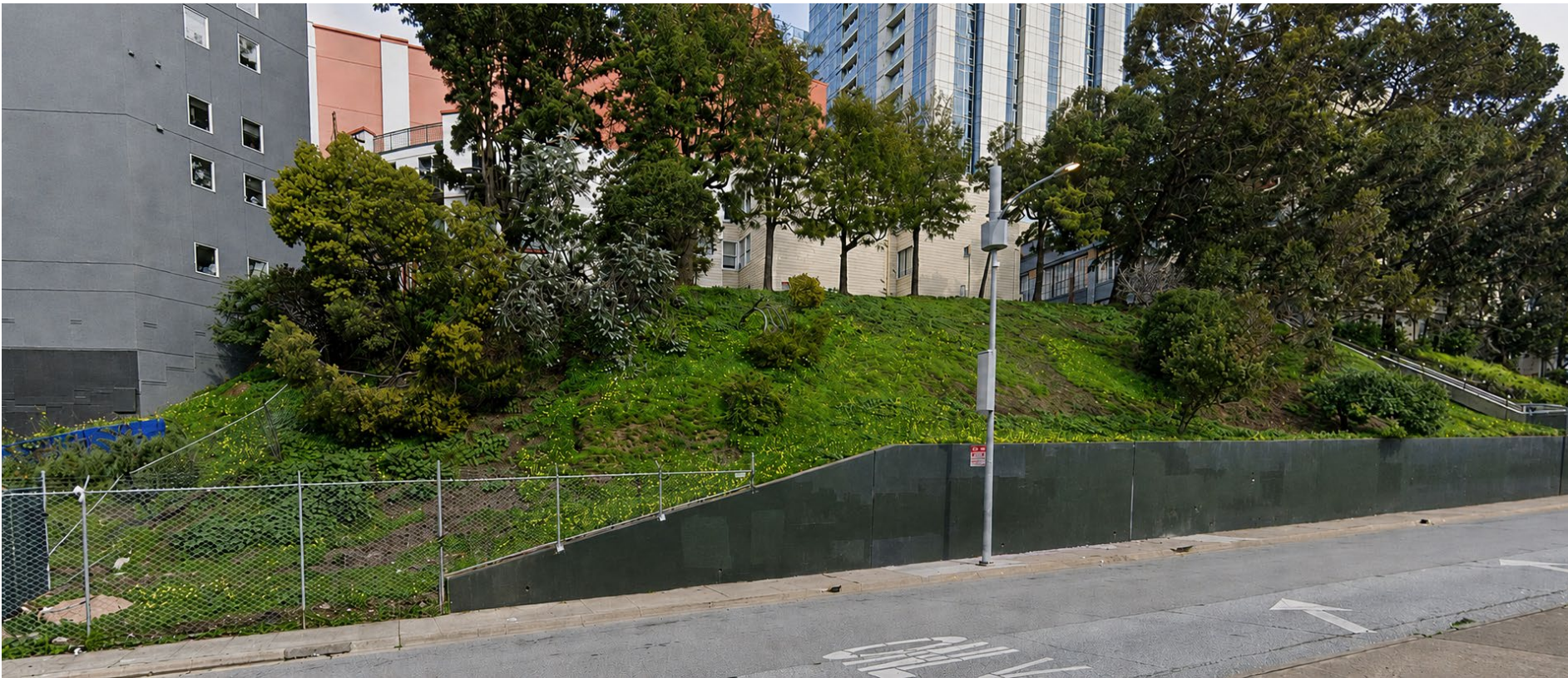
Looking at the hillside property from the Essex Street median
