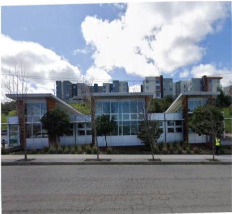
Site Office Building
