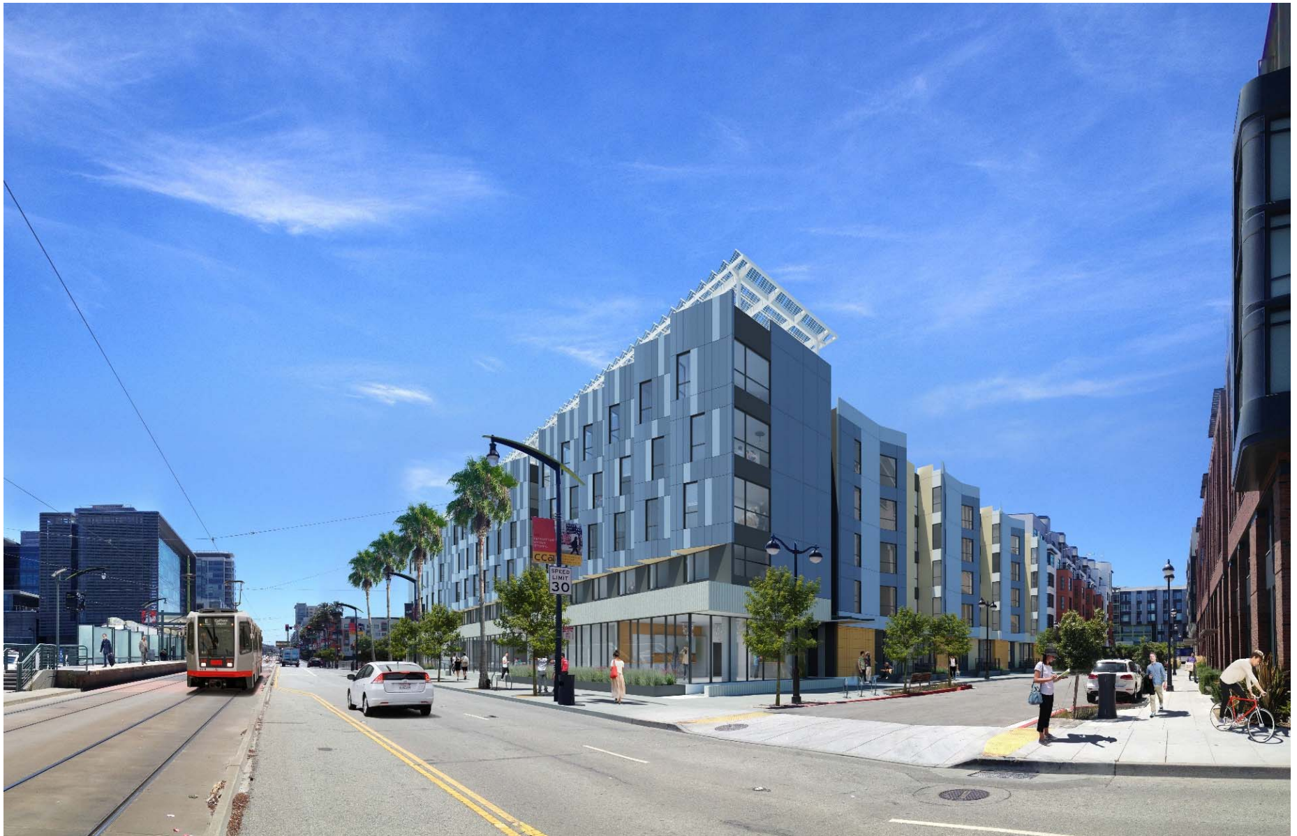
Northeast Corner from 3 rd Street & Long Bridge
